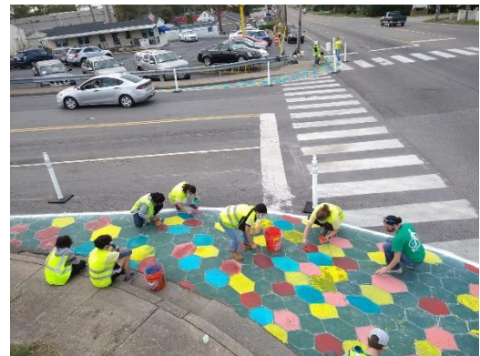
Image 3 - Nashville Youth Design Team installing bulb-outs to shorten crossing distances on Dickerson Pike, Nashville 21
