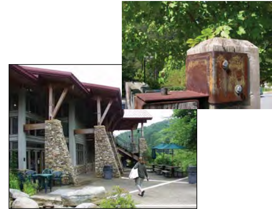
The Ocoee concept incorporates the one-sided battered stone pillar from the OWC, along with the use of dimensional exposed timbers
