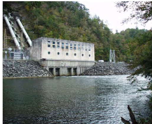
TVA Apalachia Powerhouse
