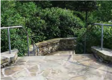
Examples of a retaining wall, steps, and guardrail
