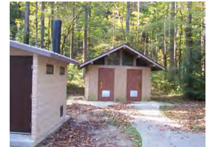
Apalachia Powerhouse River Put-In/Powerhouse
