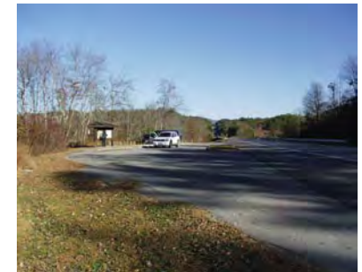
Westbound Portal Pull-off
