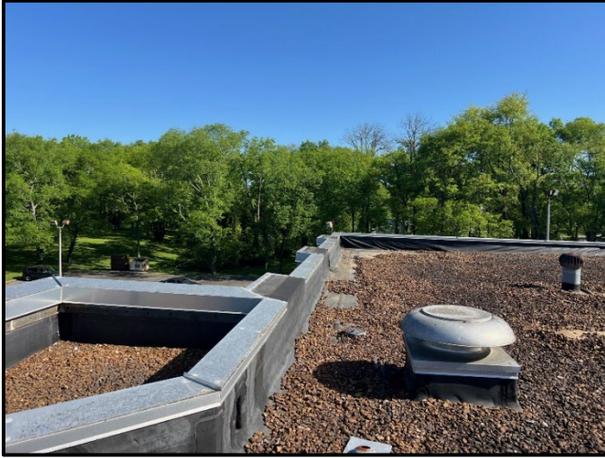
Figure 4-1: “EAST” NORTH-Facing View
