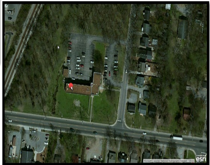
Figure 3-2: East Health Center (Aerial View)
