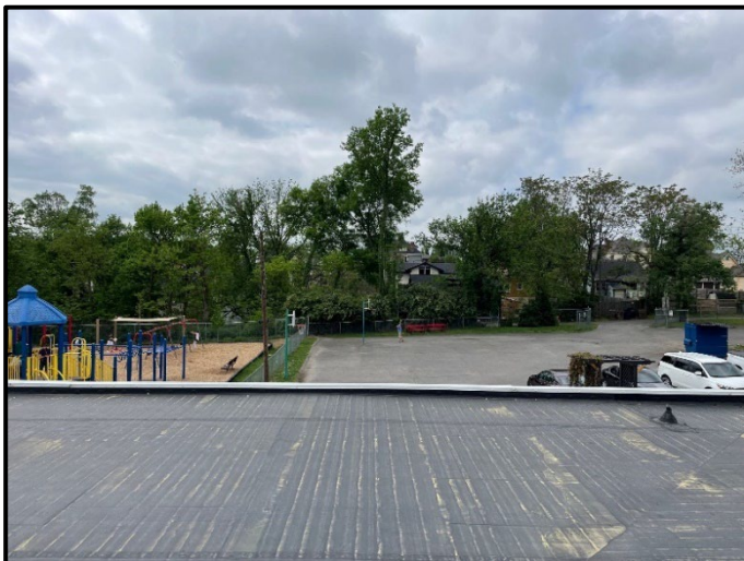
Figure 4-13: “LL” SOUTH-FACING VIEW
