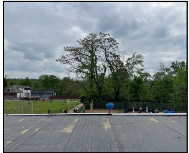
Figure 4-12: “LL” EAST-FACING VIEW
