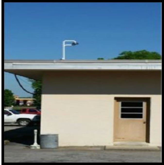
Figure 3-3: Percy Priest Dam Site
