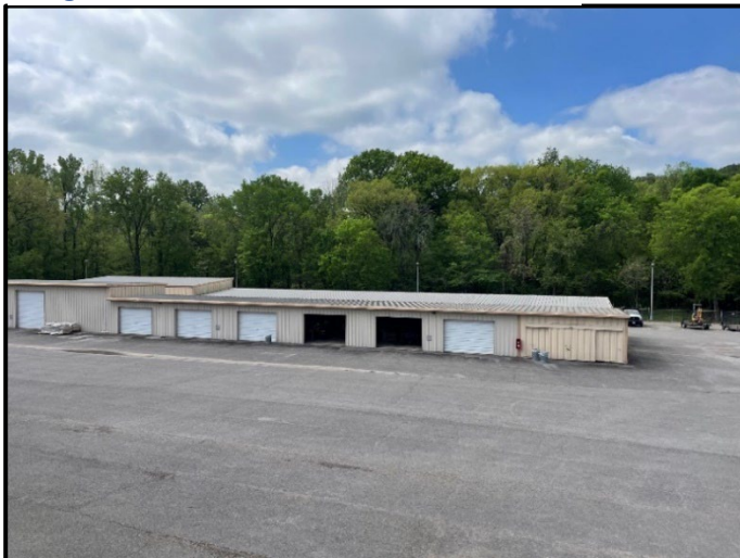
Figure 4-7: “PPD” SOUTH-FACING View
