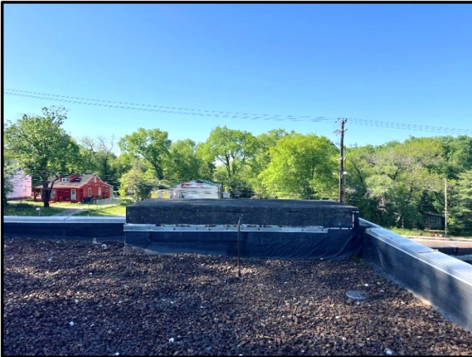
Figure 4-2: “EAST” South-Facing View
