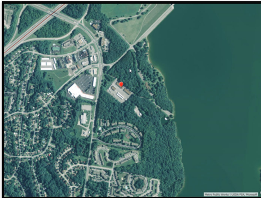
Figure 3-4: Percy Priest Dam Site (Aerial View)
