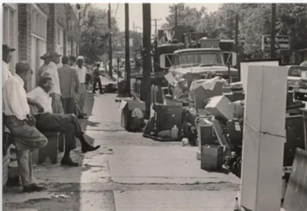
Jefferson ST residents evicted in preparation for I-40 construction
