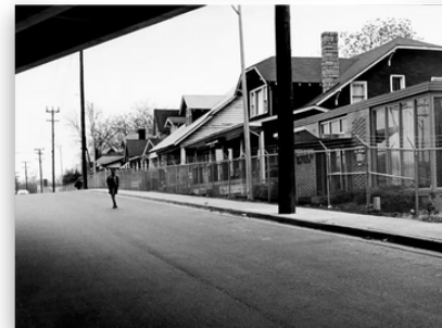
Houses and businesses along the west side of Jefferson Street are behind a 6-foot steel fence, 1970. Federal regulations require the fence be placed along ramps to the new Interstate 40
