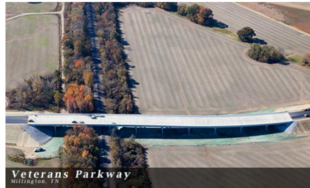
Local Programs Overpass Project (Veterans Parkway, Millington, Tennessee)
