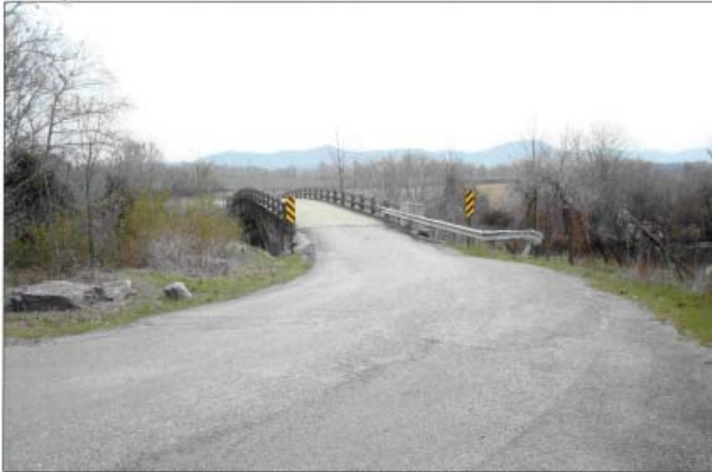
BEGIN BRIDGE APPROACH LOOKING AHEAD
