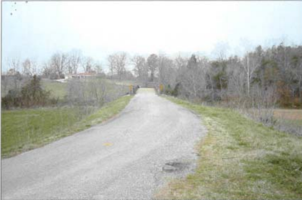
END OF BRIDGE APPROACH LOOKING BACK
