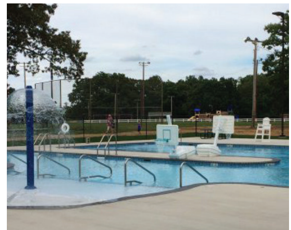
This pool was built with fly-ash concrete – a byproduct of coal combustion. It uses a recycled glass bead filter and includes other low-impact features like pervious pavement and bioswales to manage stormwater runoff in addition to high efficiency pumps and LED lighting.
