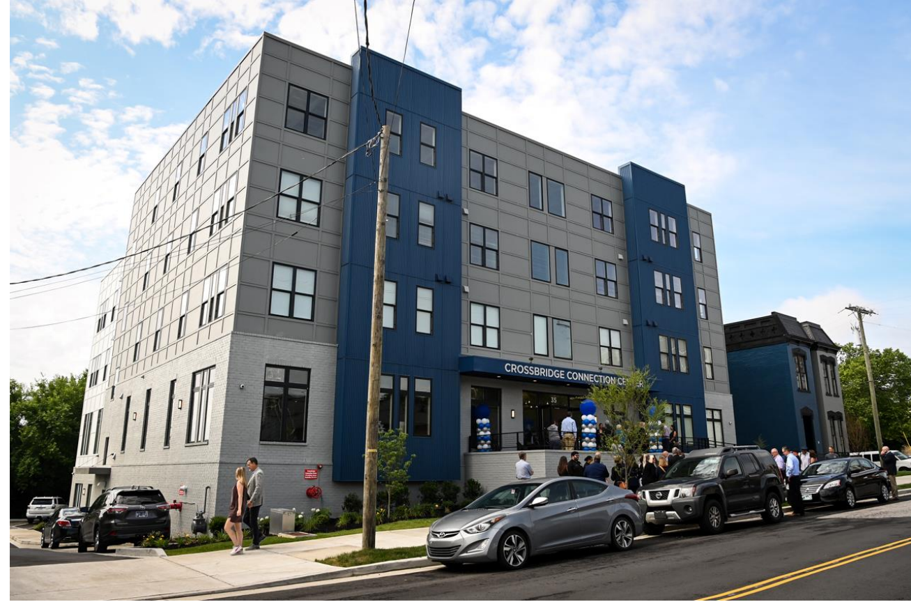
The CrossBRIDGE Connection Center in Nashville funded by CHI, Amazon, and city dollars.
