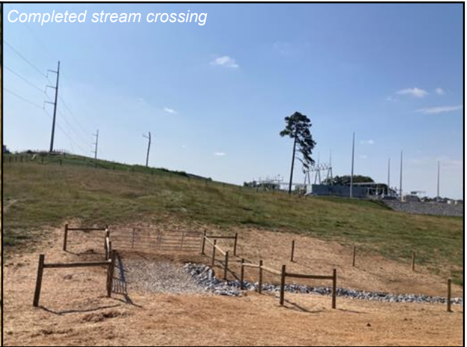
Completed rock lined outlet
