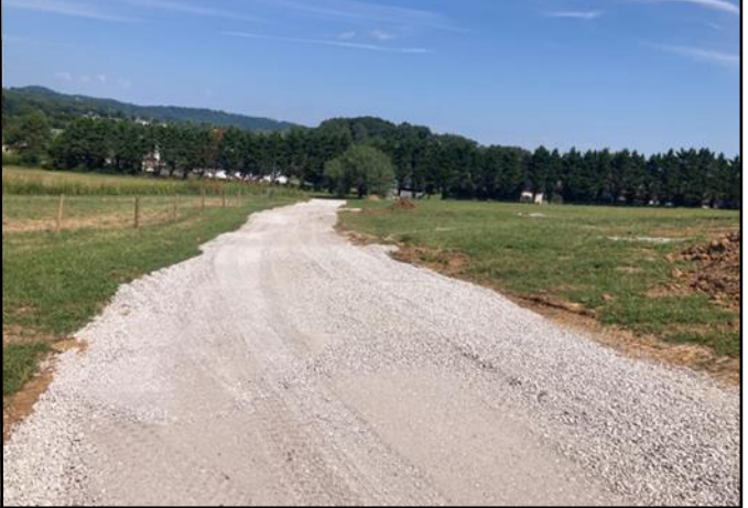
Access road project area prior to installation
