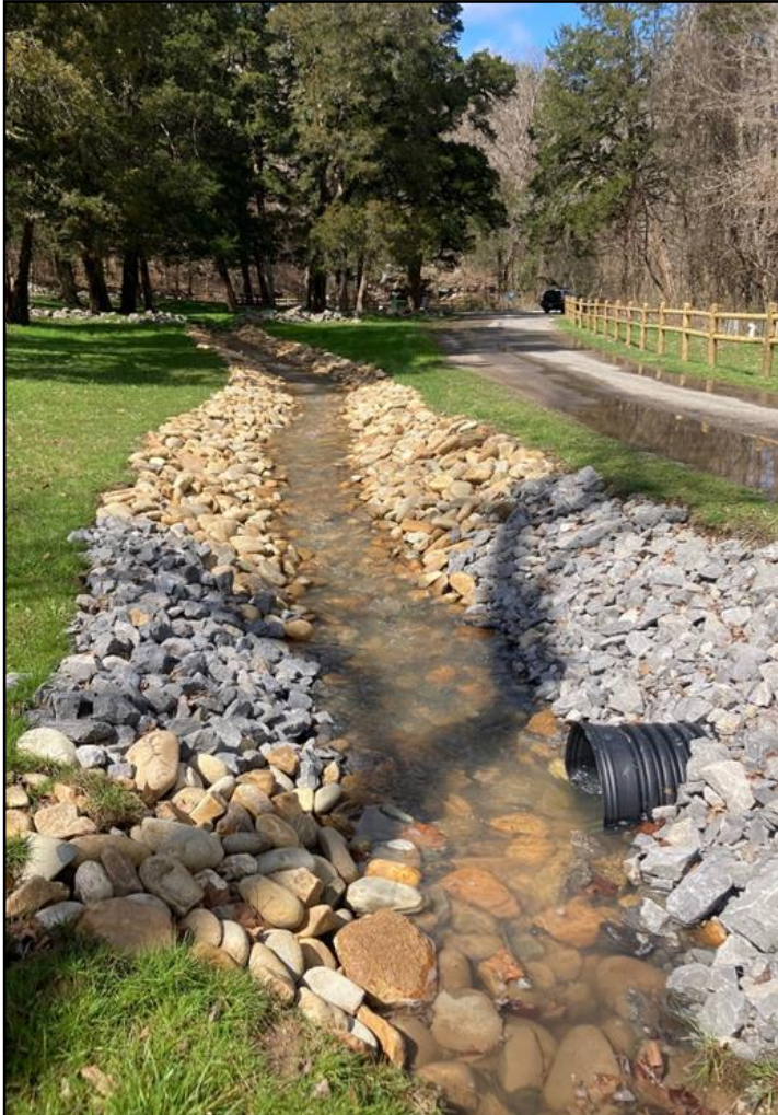
Top left: Rock armoring and culvert at "The Boils"
