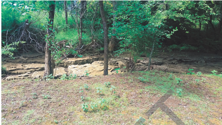
Figure 2. Lytle Creek, denuded by livestock grazing, before restoration activities in 2018.
