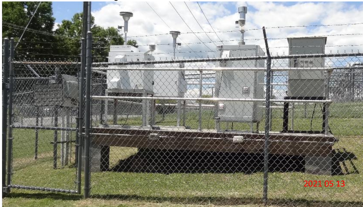
Figure 9- Deck for PM 2.5 at 911 Siskin Drive
