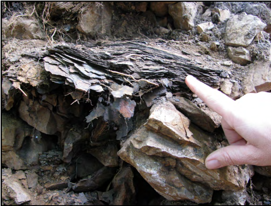
Figure 36. Trench 1, Close-up of Weathered Shale in Profile.
