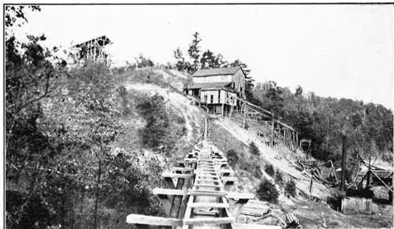
(B) Tippel, ore washer, ore bin, and waste flume at Aetna brown iron ore mine of former Bon Air Coal & Iron Corporation, 1921.
