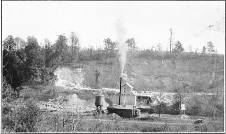
(A) Fluxing-limestone quarry and crushing plant of the former Bon Air Coal & Iron Corporation, half a mile south of Wrigley furnace.
