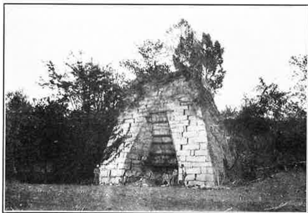
(B) Stack of Vernon furnace near Eaton flag stop, Montgomery County.
