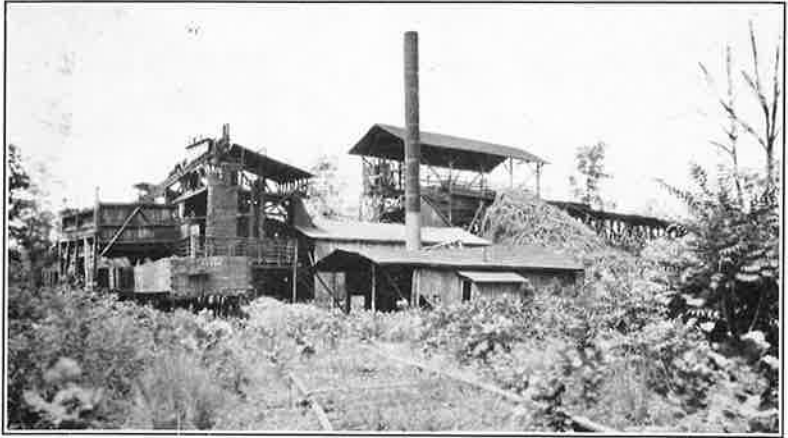
(A) Washing plant at Iron Hill brown iron ore mine, Dickson County, August, 1927.
