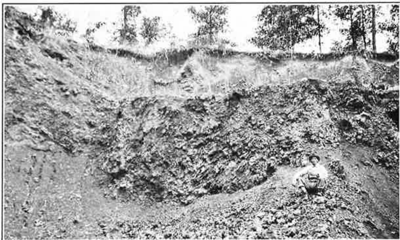
(B) Cut in Aetna brown iron ore mine, showing deposit of high-grade ore behind J. T. Brown, Superintendent.
