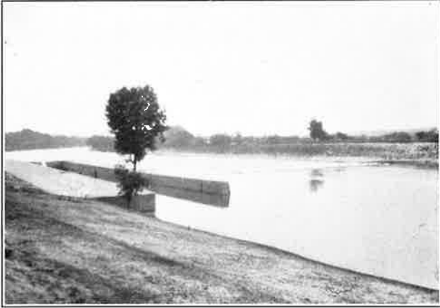
(A) Lock D on Cumberland River just below Dover, Stewart County, 1923.
