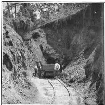
(A) Active cut at Louise mine, Montgomery County, 1923.
