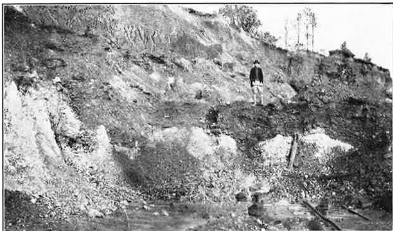
(A) Cut in Aetna brown iron ore mine, showing ore overlying white clay.
