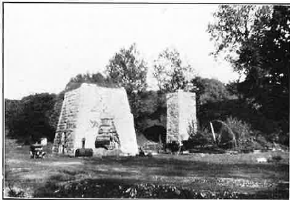
(B) Stack of Bear Spring furnace at Bear Spring, Stewart County, erected 1873.
