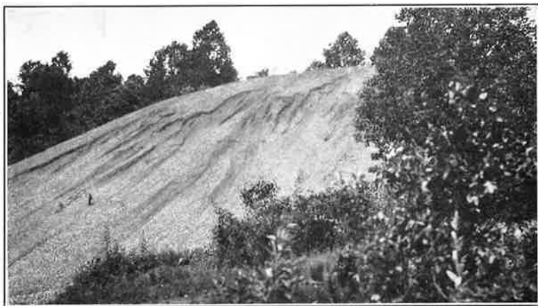
(B) Waste pile of chert and limonite discharged from washers at Pinkney brown iron ore mine, Lawrence County, 1923.
