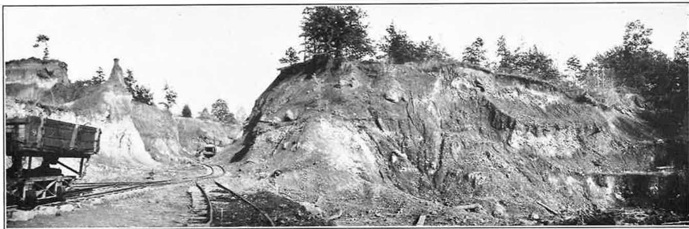
(B) Main cut in Aetna brown iron ore mine, Hickman County, 1921.
