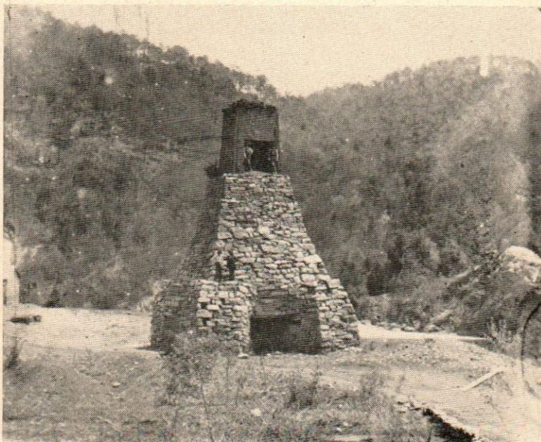
Charcoal-burning furnace on Nolichucky River, one mile below Embreeville. Furnace erected in 1861 or earlier, destroyed by flood in 1901. Photograph taken in 1885 by J. M. Fink, published by courtesy of Paul M. Fink.
