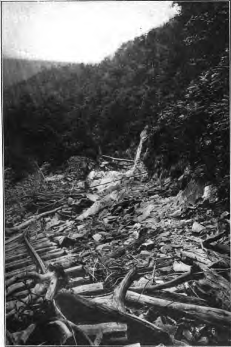
FLOOD DAMAGE TO RAILWAY ON NOLICHUCKY RIVER, MAY, 1901—UNICOI COUNTY.
