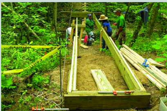
Start of the Beaman Park Trail Bridge Project, building the main beams
