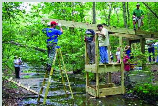
Start of the Beaman Park Trail Bridge Project, building the main beams across the creek.
