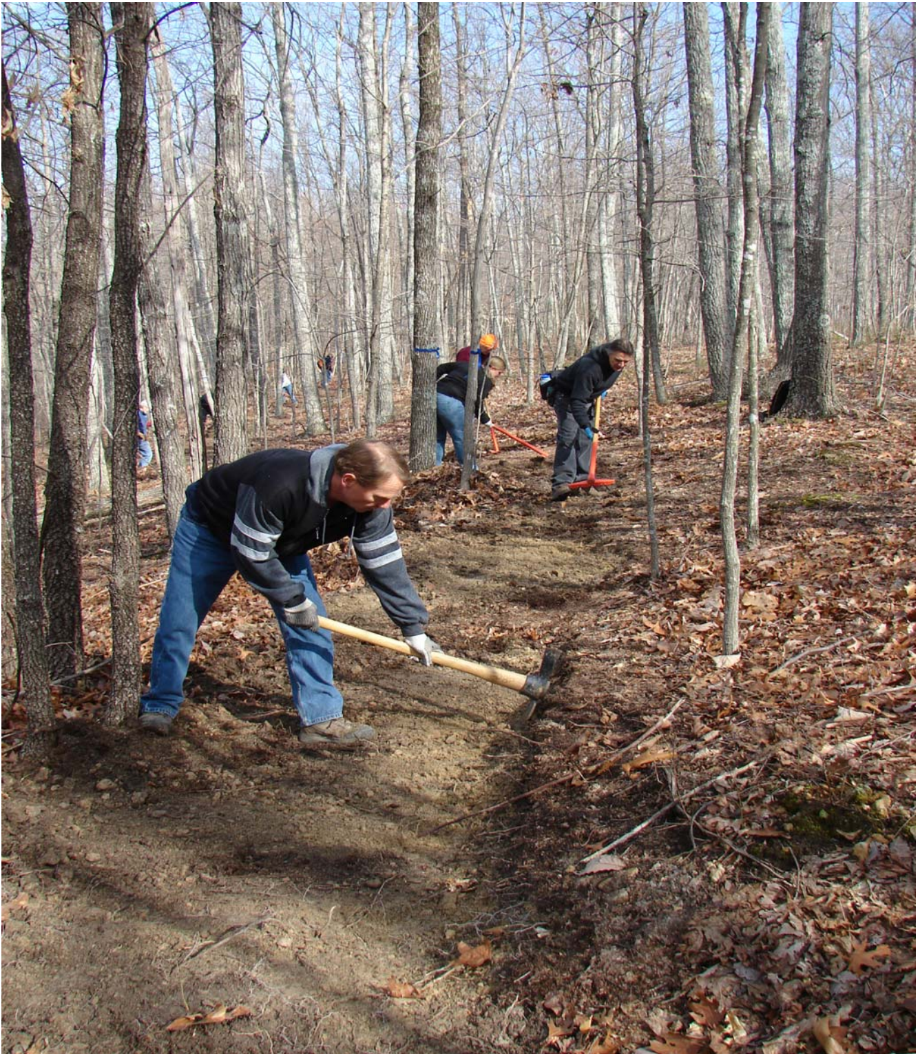
Cutting the back slope on a graded section of trail
