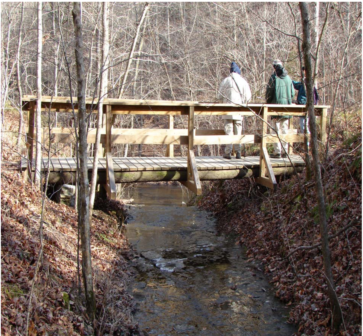
20' trail bridge at Beaman Park
