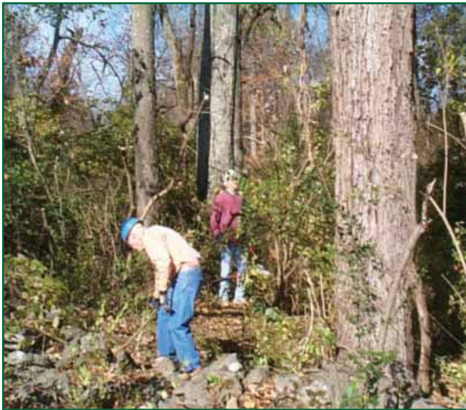
Building the trail using hand tools
