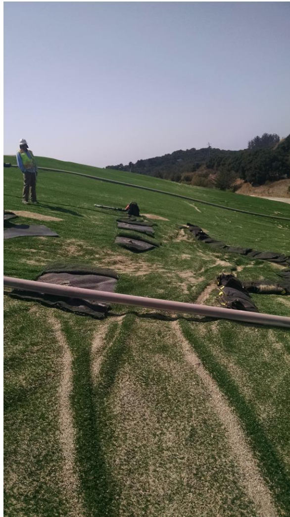
Repair of Depression Area on a Landfill Final Cover Side Slope
