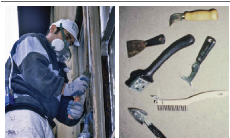
FIGURE 12.16 Wet scraping (left) FIGURE 12.17 Scraping tools (right).
