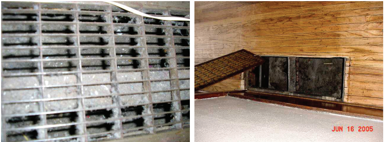
Figure 11.24 Air vent before and after cleaning.
