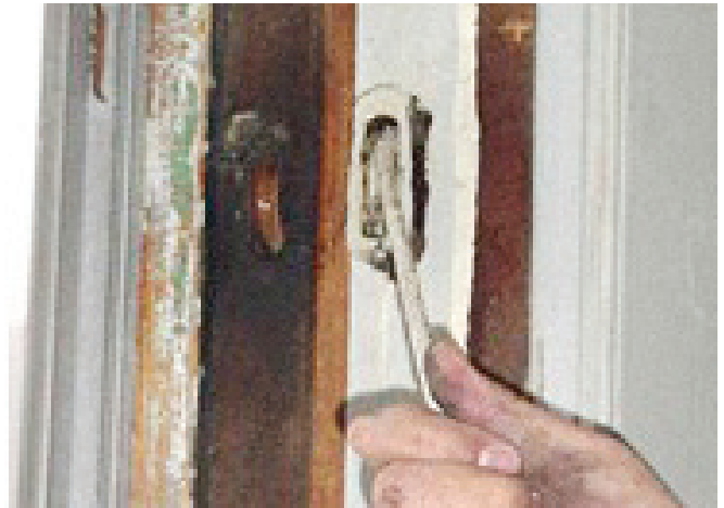
FIGURE 11.8 Remove sash controls/weights.
