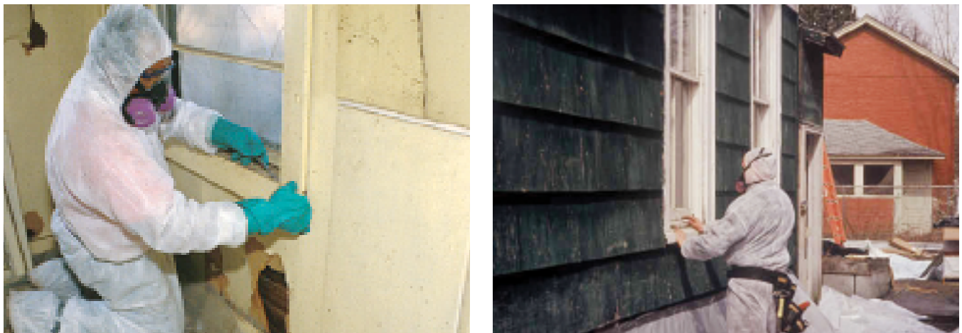
FIGURE 12.1 Removing and Replacing Trim: interior (left), exterior (right).
