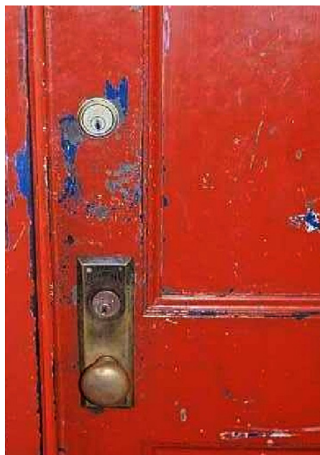
FIGURE 1.3 Paint deterioration.
