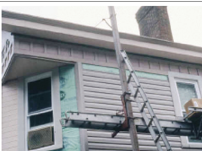
FIGURE 12.6 Installation of replacement siding.
