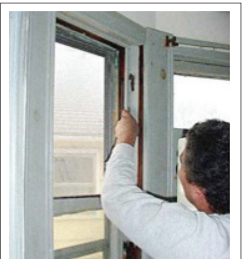
FIGURE 11.6 Remove parting Ahead.
