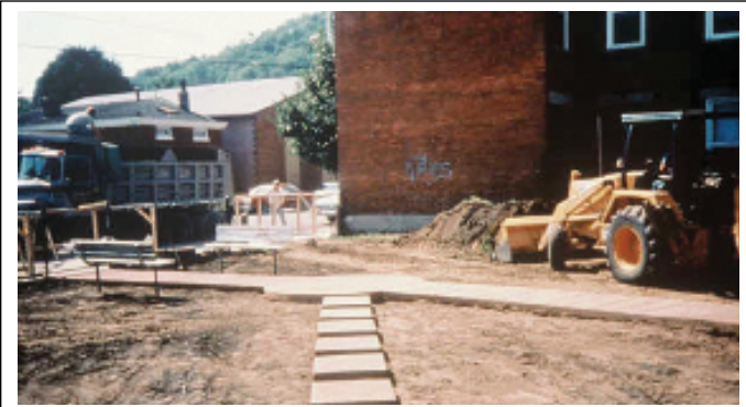
FIGURE 12.22 Replacing resident pathway after soil removal.
