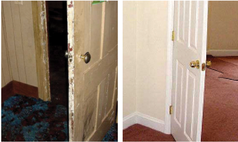
FIGURE 12.4 Pre-and post-abatement interior doors.
