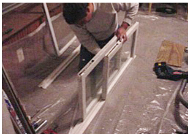
Figure 11.13 Fit sashes into jamb liners.
