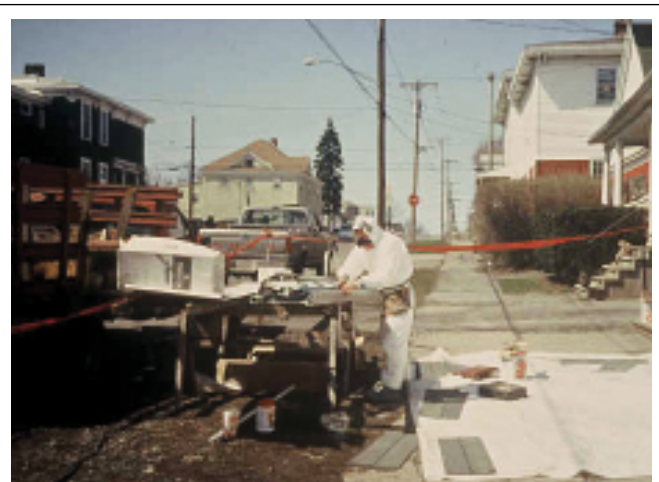
FIGURE 12.7 Certified workers are needed to replace siding when the project's intent is lead abatement.
