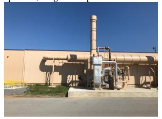
"We have what is known as a Regenerative Thermal Oxidizer unit to collect and control air emissions from the testing of our fuel injection products," said Eddie Franks, Supervisor for Safety Health and Environment at DMAT. "We are upgrading that system to become an energy source for us." The typical thermal oxidizer system captures and destroys volatile organics like the fuel used for the final testing for each fuel injector that DMAT manufactures. The new system would
