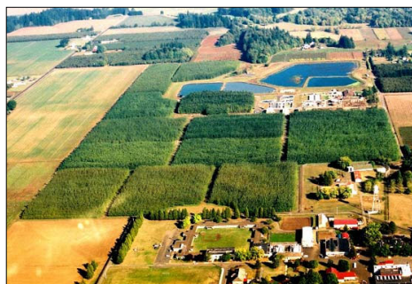
Wastewater Treatment Plant & Poplar Tree Reuse System; Woodburn, Oregon
