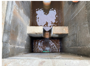
Triangular (V-notch) Weirs
