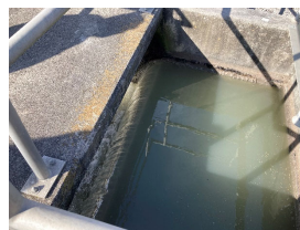
Rectangular Weir without end constrictions
