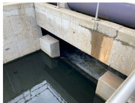
Rectangular Weir with end constrictions
