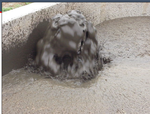
Waste Activated Sludge Systems
