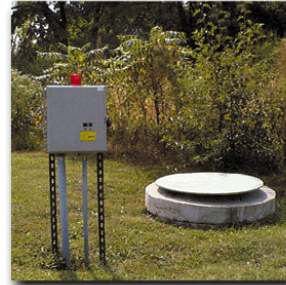
Submersible lift stations are designed to blend readily with natural surroundings, since there is no pump house and there is a minimum of above-ground equipment. Other advantages to below-ground installations are noise reductions and less safety-hazard concerns.
