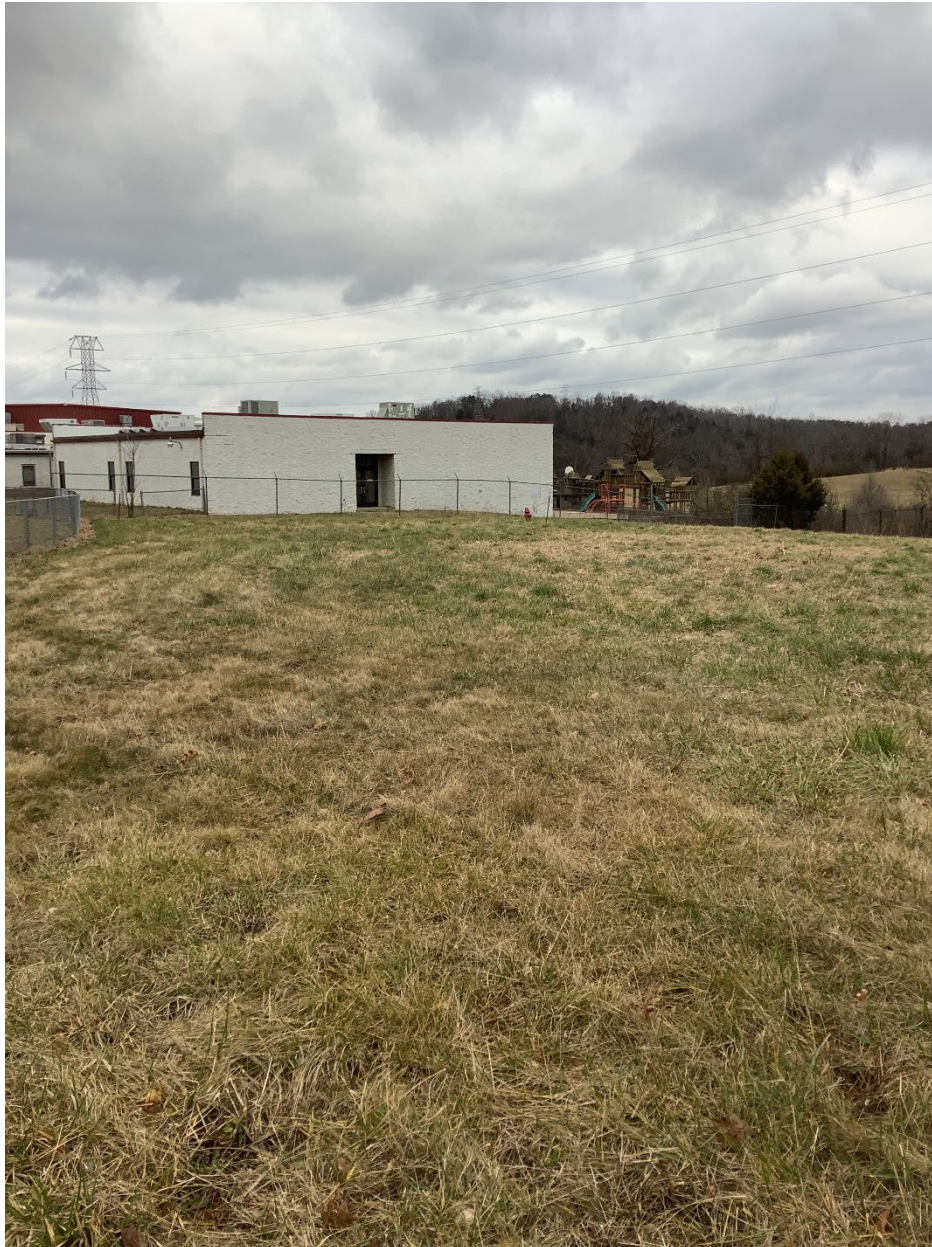
A1. No apparent drip field overload or other malfunction.
