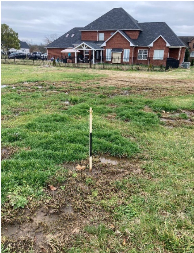
Photo 1. Dysfunctional Land Application Area
