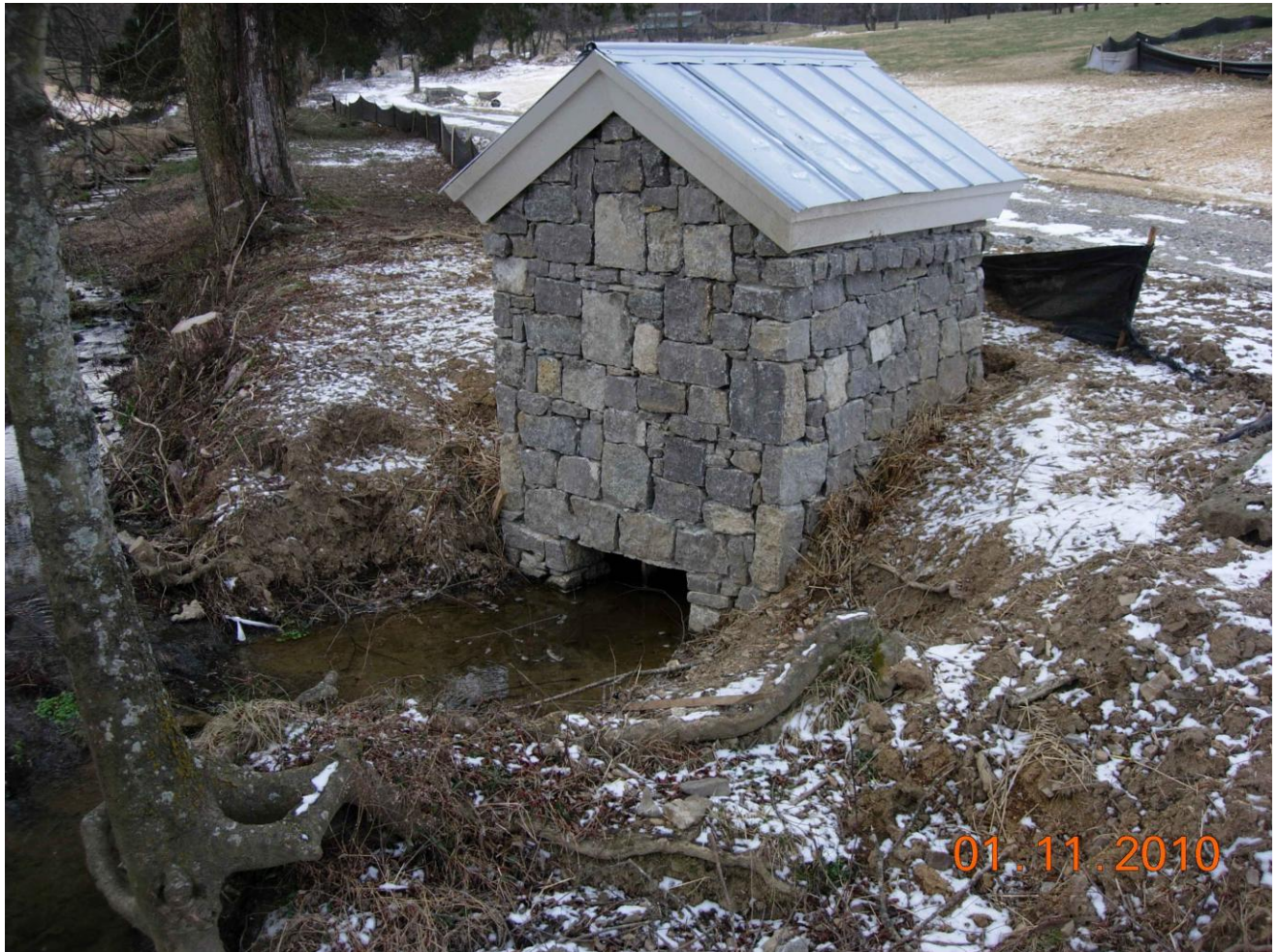
Figure 3. Springbox (newly restored)
