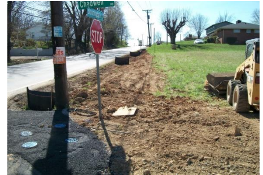
Bloomington Utility District's Waterline Replacement $2.5M
