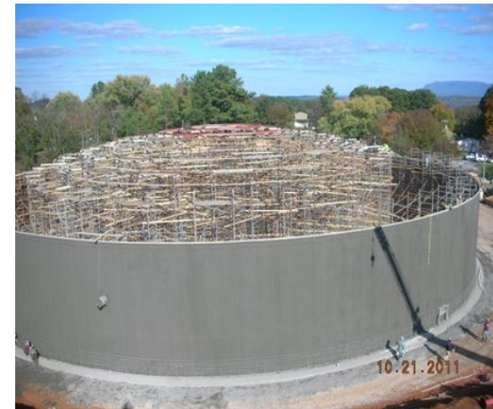
Alcoa Overlook Water Storage Tank $5M
