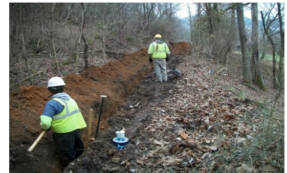
Elizabethton Waterline Replacement $650K
