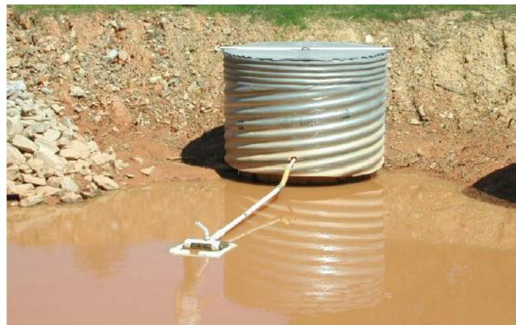
Figure 7.31-10B Floating Skimmer Installation
