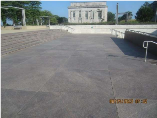
Overview of the 3 rd Floor Plaza above the entrance area. NRC anticipates a waterproofing to be installed below the finish surface. Drainage locations are recommended to be observed closely.
