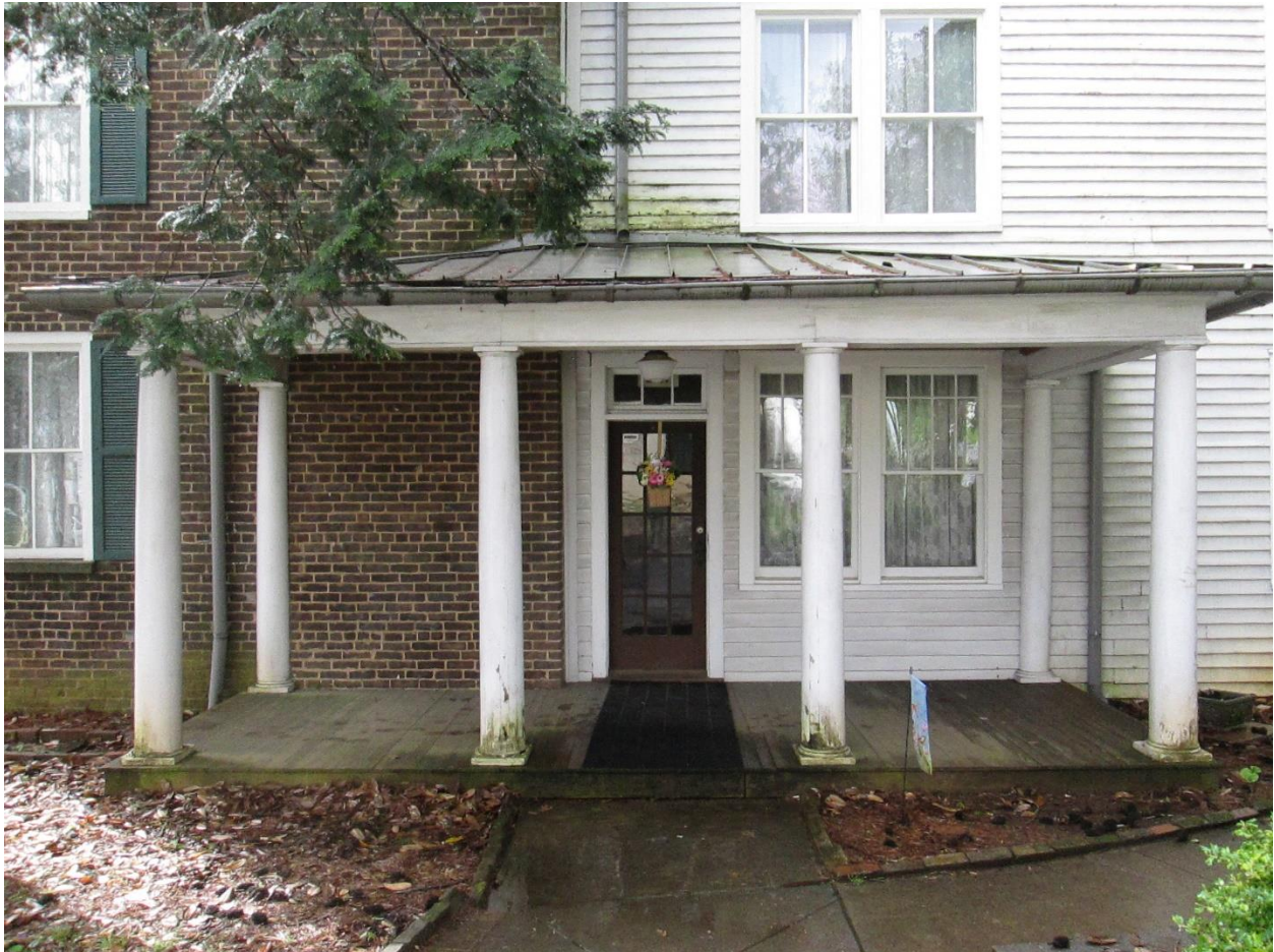
Photograph 4. Partial view of the north elevation of the Nance Building, facing south, showing the entire porch including the four freestanding columns and two pilasters.
