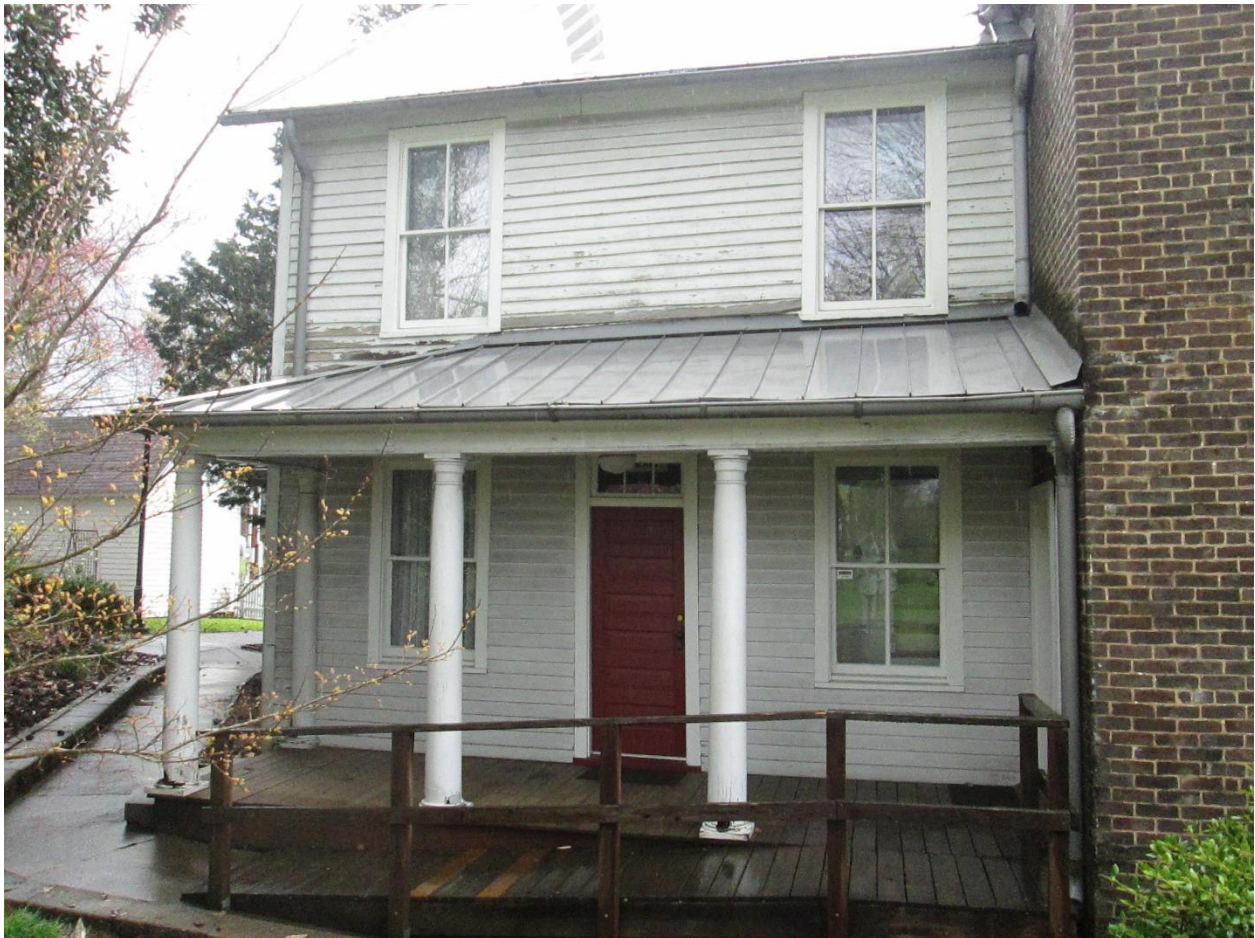
Photograph 1. Partial view of the west elevation of the Nance Building, facing east, showing the entire porch including the three freestanding columns and two pilasters.
