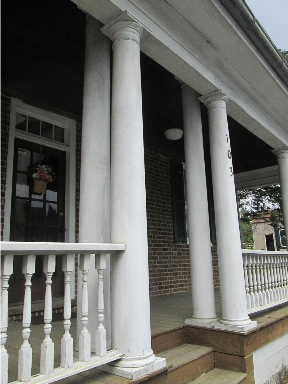
Photograph 8. Examples of the freestanding columns along the east elevation (façade) of the Nance Building, shown in fair condition.
