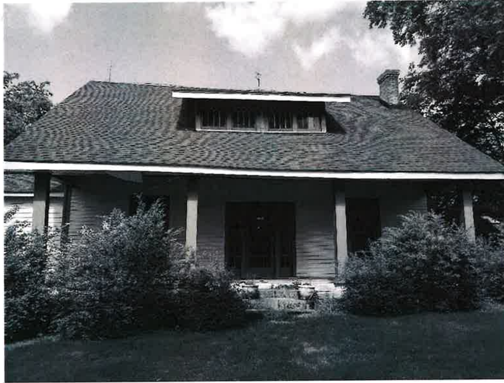
Ford House Structural Inspection
