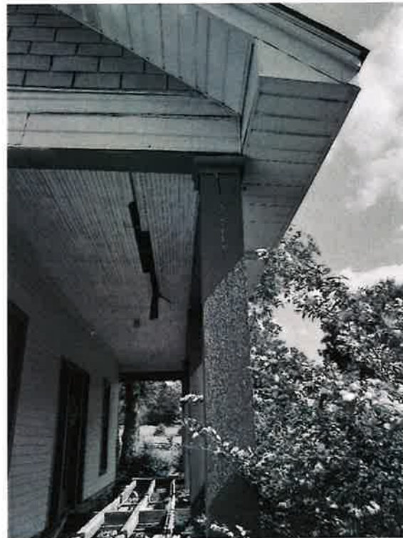
Photo No. 14. South column of porch framing.
