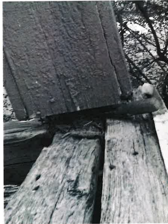
Photo No. 15. Base at south column of porch framing.
