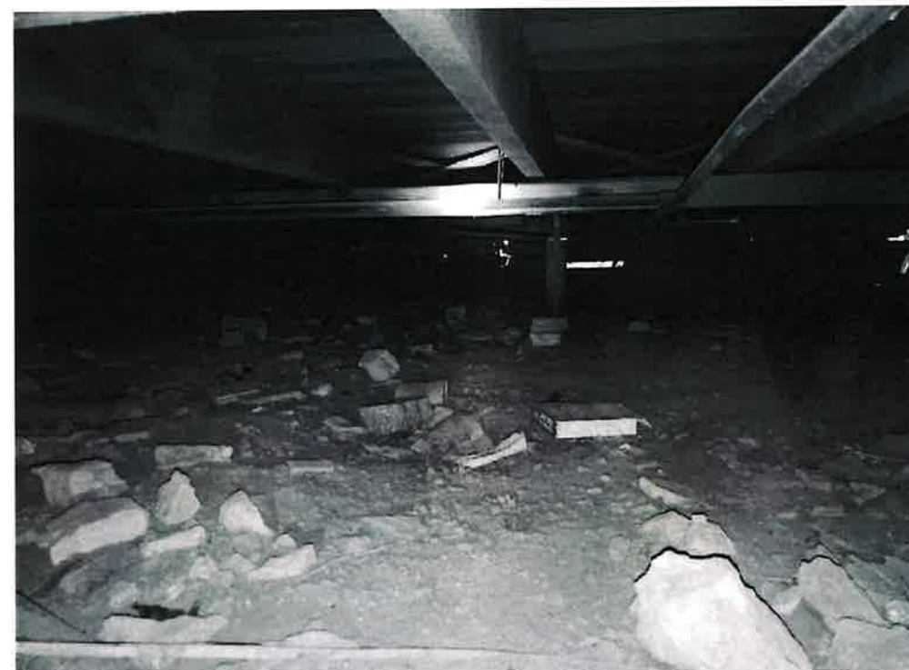
Photo. No. 18. Cantilever rehabilitation support with small foundation.
