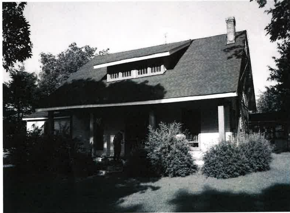
Photo No. 1. Overall building.
