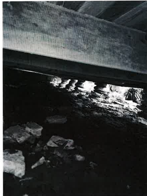
Photo No. 8. Individual stone piers on east portion of building.
