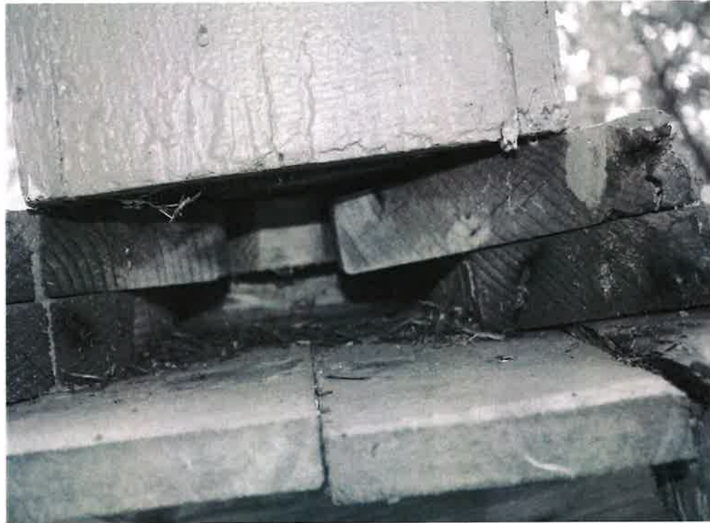
Photo No. 13. Closeup of column base.
