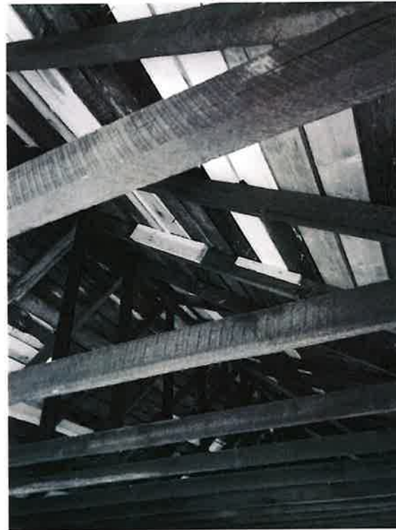
Photo No. 19. Typical truss chord rehabilitation.
