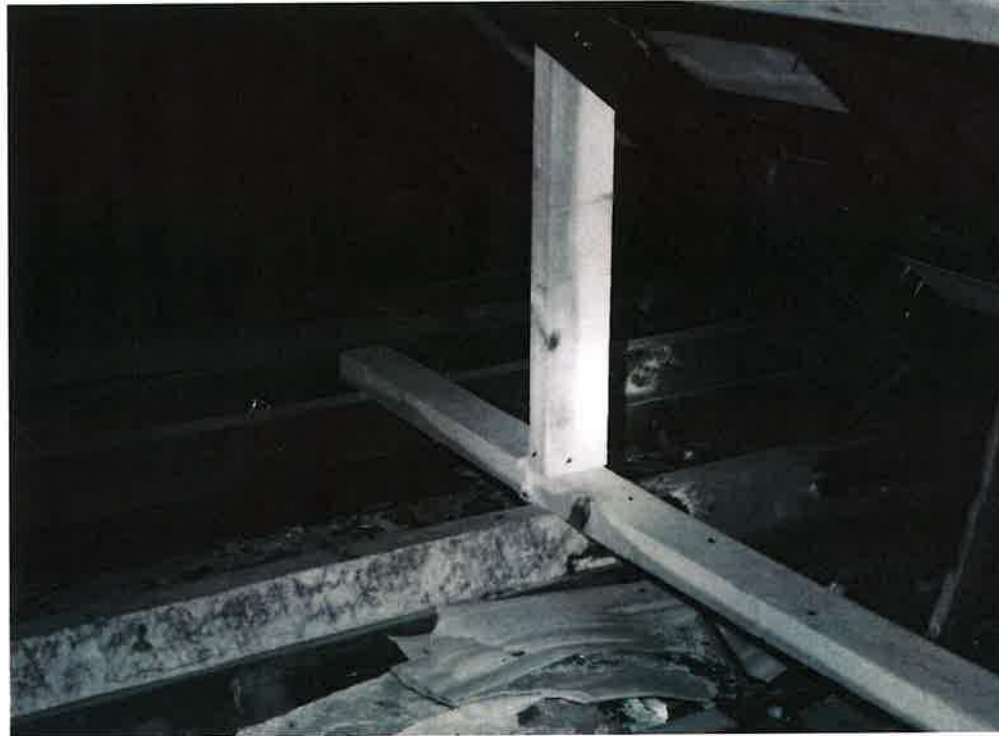
Photo No. 25. Rehabilitation framing with redistribution of load.
