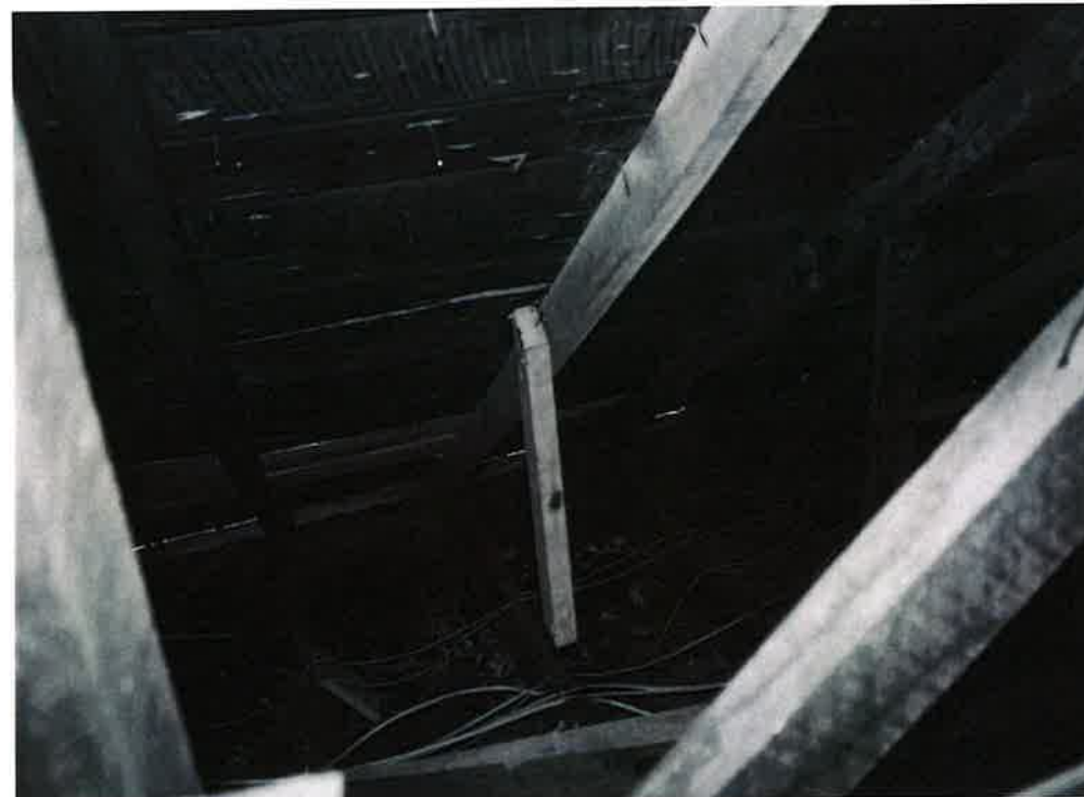
Photo No. 22. Connections at bracing with gaps.
