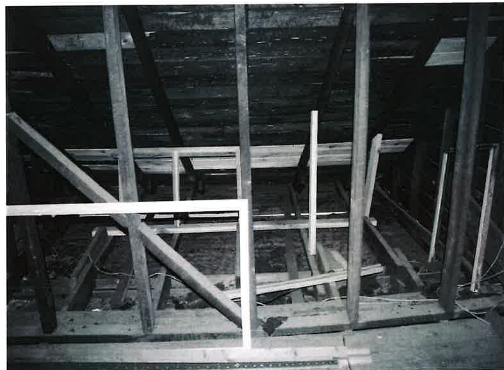
Photo No. 20. Truss rehabilitation with differential load path.
