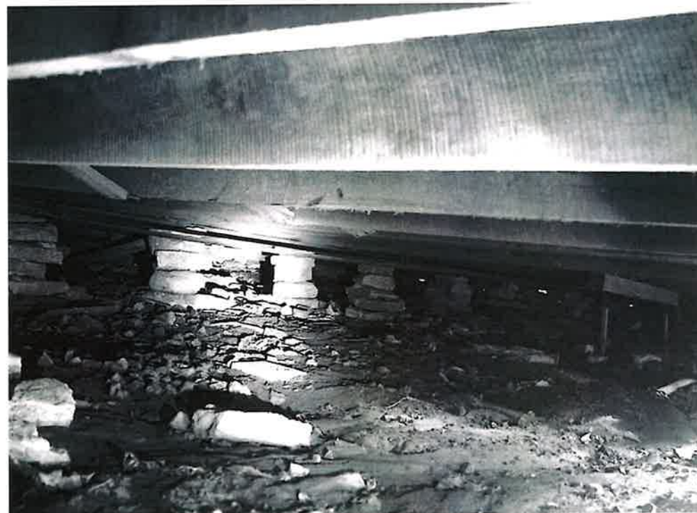
Photo No. 4. Individual stone piers at interior support.
