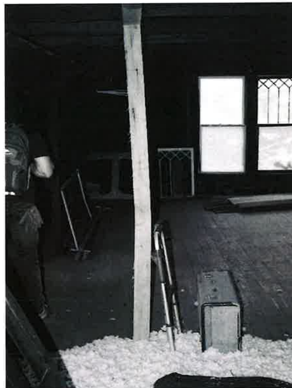
Photo No. 30. Rehabilitation frame for attic truss that redistributes load path.
