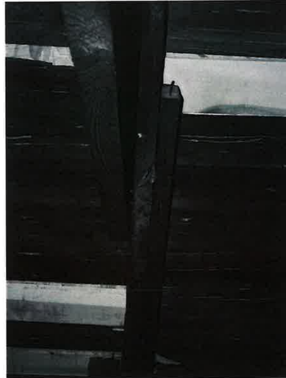
Photo No. 26. Gap at connections of roof trusses.
