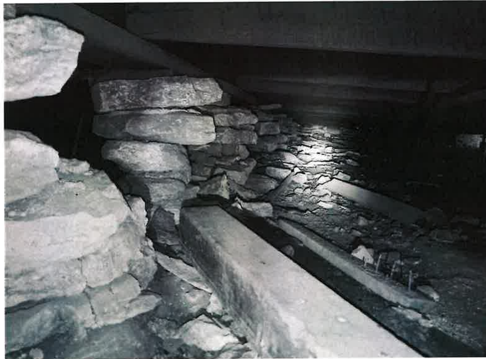
Photo No. 5. Individual stone pier foundation at interior support.
