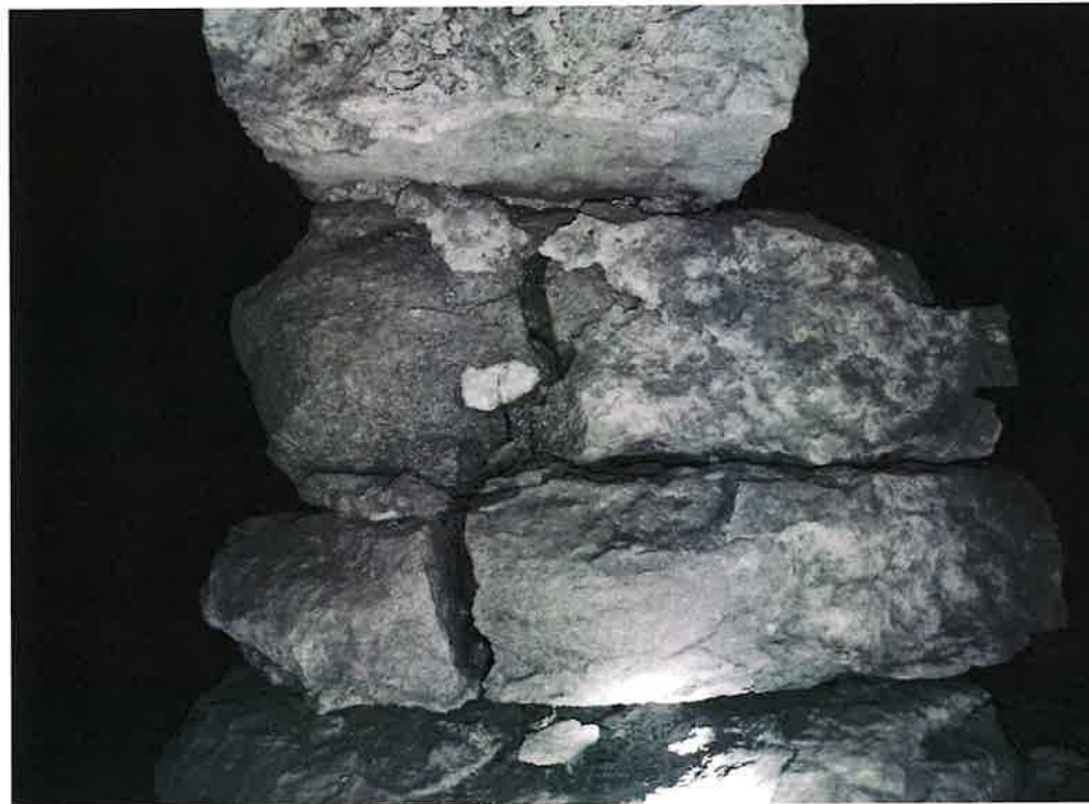
Photo No. 9. Cracks developed in stone pier.
