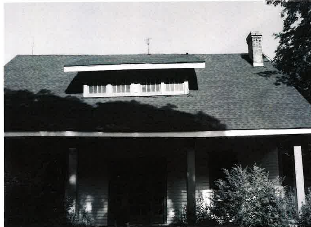
Photo No. 2. Exterior east elevation.
