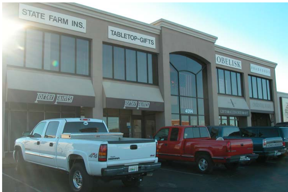
FIGURE 3 - Photo of the storefront, Bradford Building, 4094 Hillsboro Pike. Nashville, Davidson County, Tennessee. (Photo credit: David Borowski, TDH, 12/20/04)
