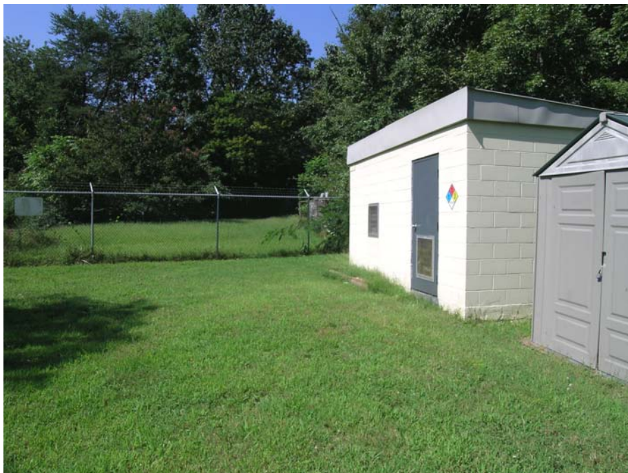
FIGURE 3 - Photo of the well building at the WRUD water treatment facility. The tetrachloroethylene spill occurred on the property beyond fence; approximately 100 yards from the well building. Hamilton County, Tennessee. (Photo credit: Ron Clendening, TDH, 8/31/05)
