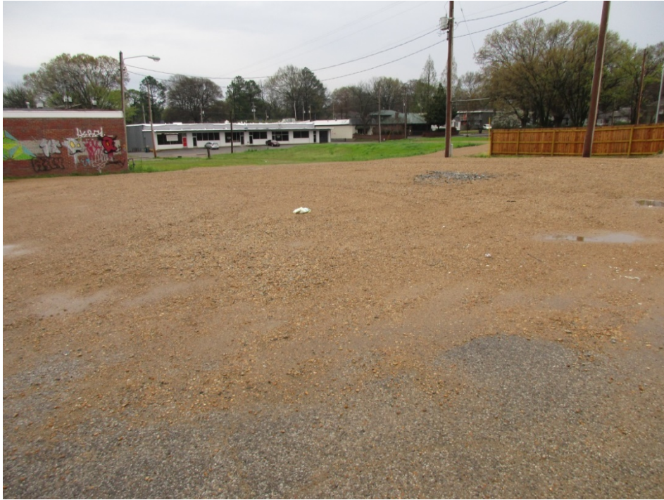
Photo 3 – Former Custom Cleaners/Sharri’s Discount Art Supplies building location. After building demolition and soil removal, gravel was part of the fill material brought onto site to fill the source area soil excavation. View is to the southeast toward nearby business strip center housing a rug cleaning company and vacant storefronts on Minor Road. (Photo credit: J. George, 3/27/17).
