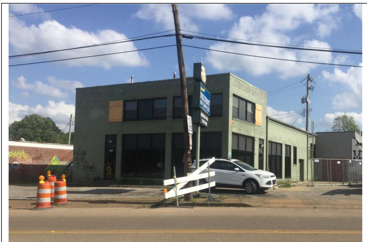
Figure 2. The Former Custom Cleaners building, which formerly housed Sharri's Discount Arts. Southern Avenue is in the foreground. The dry-cleaning machine was located in the back left of the building. View is looking south. [Photo credit: J. George, TDH, 4/26/16].
