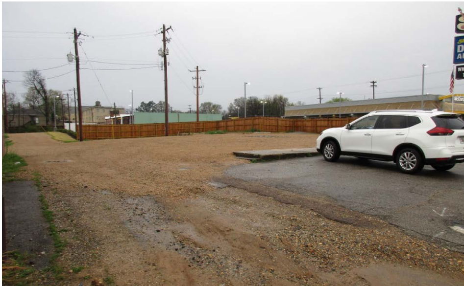
Photo 4 – Former Custom Cleaners building location after EPA emergency response action. EPA removed source area soil to a depth of 17 feet from beneath the FCC building in 2016. View is looking southwest. (Photo credit: J. George, TDH, 3/27/17).
