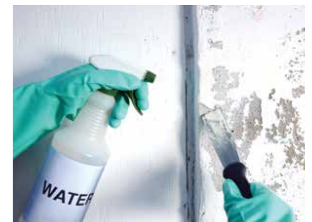
PHOTO: Wet-misting lead paint reduces dust hazard.
