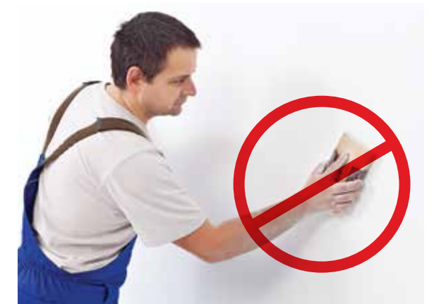
PHOTO: Do NOT sand lead paint. Use removal methods that control dust.
