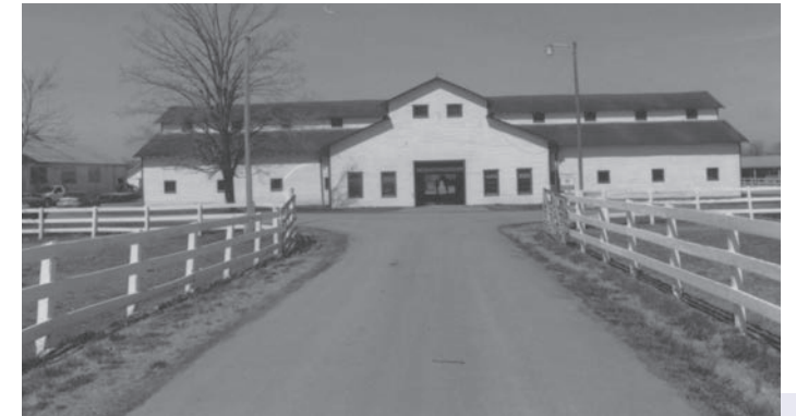
The Main Horse Stable at Harlinsdale Farm in Franklin, Williamson County is a great example of a monitor roof barn. Constructed in 1935, this barn was the centerpiece of the Harlinsdale Farm, a property nationally known for its superior Tennessee Walking Horses. The Farm was listed in the National Register on May 3rd, 2005. Photograph courtesy of Carroll Van West, 2005.
