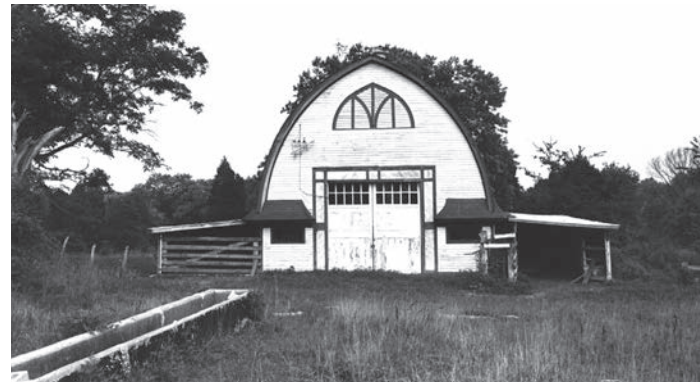
This fine Gothic Roof barn is located on the National Register-listed Milky Way farm in Pulaski, Giles County. It is likely the barn was constructed in the 1930s. The gothic arch, windows, and entry speak to a high attention to detail. The farm was listed in the National Register on September 27, 1984. Photograph courtesy of Kim Chiles, May 1984.
