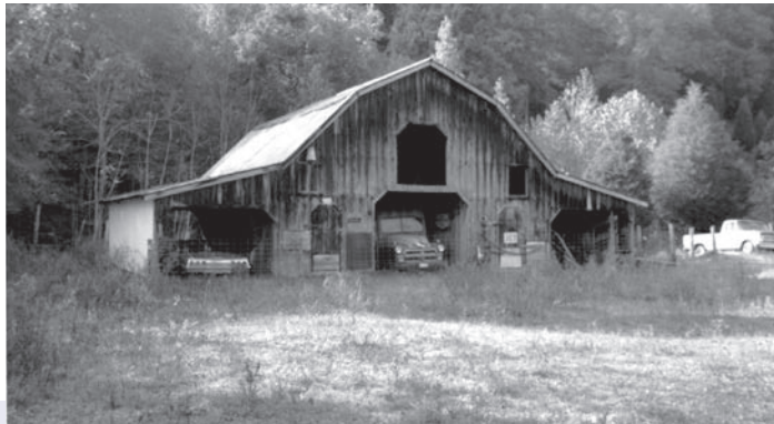
The Craig Family Farm (National Register-listed May 15, 2006) barn is a good example of a Central Aisle Barn. Constructed by McDonald Craig in 1970, the barn housed livestock and the school bus Craig used to drive local African American students to school during segregation. The flexibility of these barn types ensured their continued use and preservation on the rural landscape. Photograph courtesy of Caneta Hankins, 2004.
