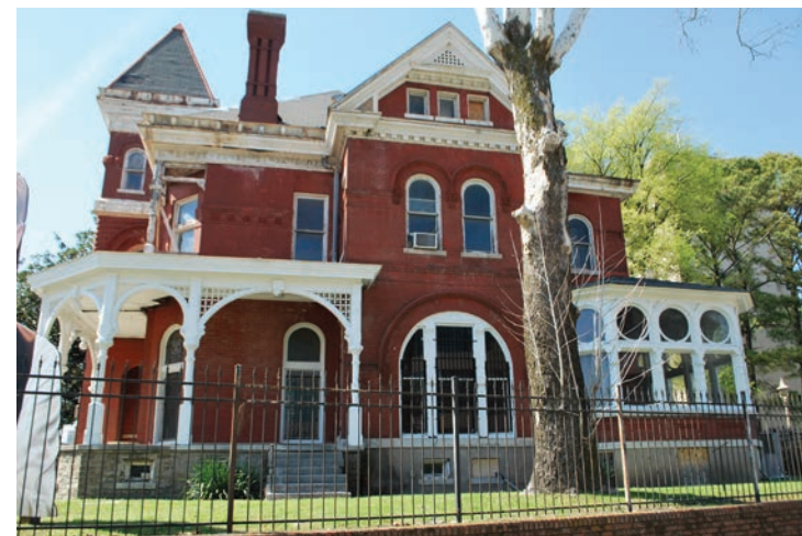
Side elevation view of the Lowenstein House.
