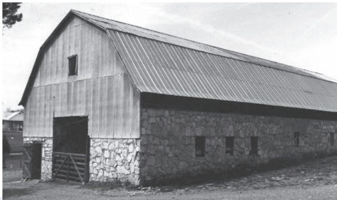
The Bradford Rymer barn is both an excellent example of a Gambrel roof and a rock barn. Built in 1930 by Bradford Rymer, it is a two-story Central Aisle Barn constructed entirely of stone and capped with a metal Gambrel Roof. At the time of survey, it was the only stone barn in Meigs County. The Bradford Rymer Barn was listed in the National Register of Historic Places on July 6, 1982. Photograph Courtesy of Stephen T. Rogers, November 26, 1980.
