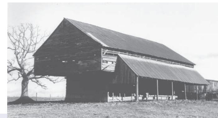
The Carl Trundle Barn was constructed ca. 1900 by John Keller and listed in the National Register on July 25, 1989. It is a rectangular Cantilever barn with two log pens separated by a central runway. The logs are joined using half dovetail notching, and the interior bracing is mortise and tenon construction. Photograph courtesy of Philip Thomason, March 30, 1989.
