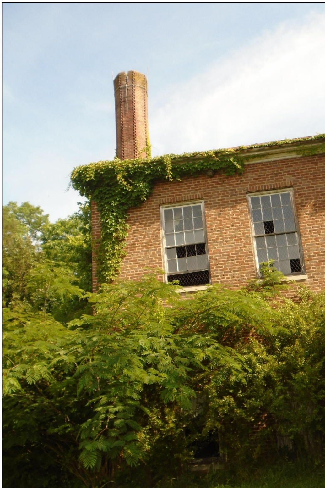
Figure 4: Circular Chimney on the West Wing, June 2020
