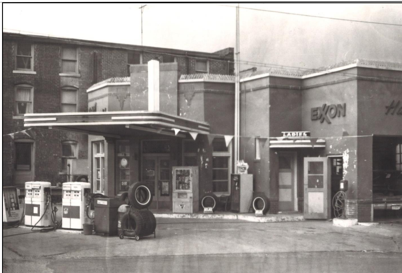
Figure 2: 1978 Survey Photo of the Esso Filling Station. From the Tennessee Historical Commission.
