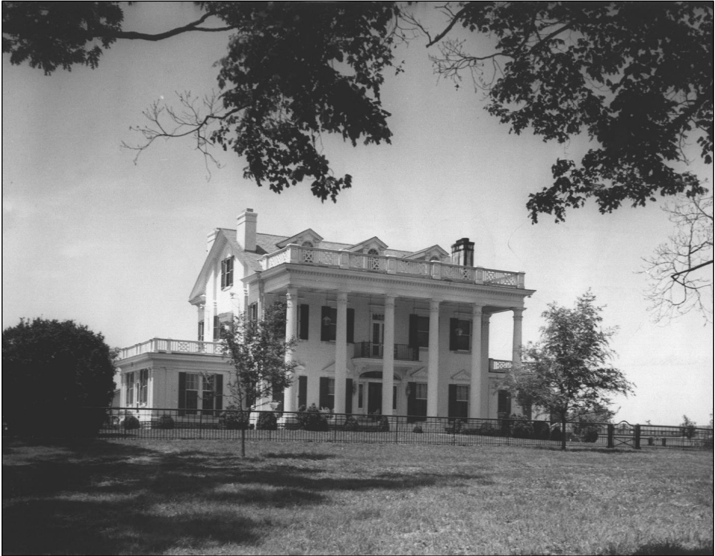
Figure 22: John L. Haynes House, Haynes Haven Stock Farm, 1940. Tennessee State Library and Archives, Department of Conservation Photograph Collection, 1937-1976.
