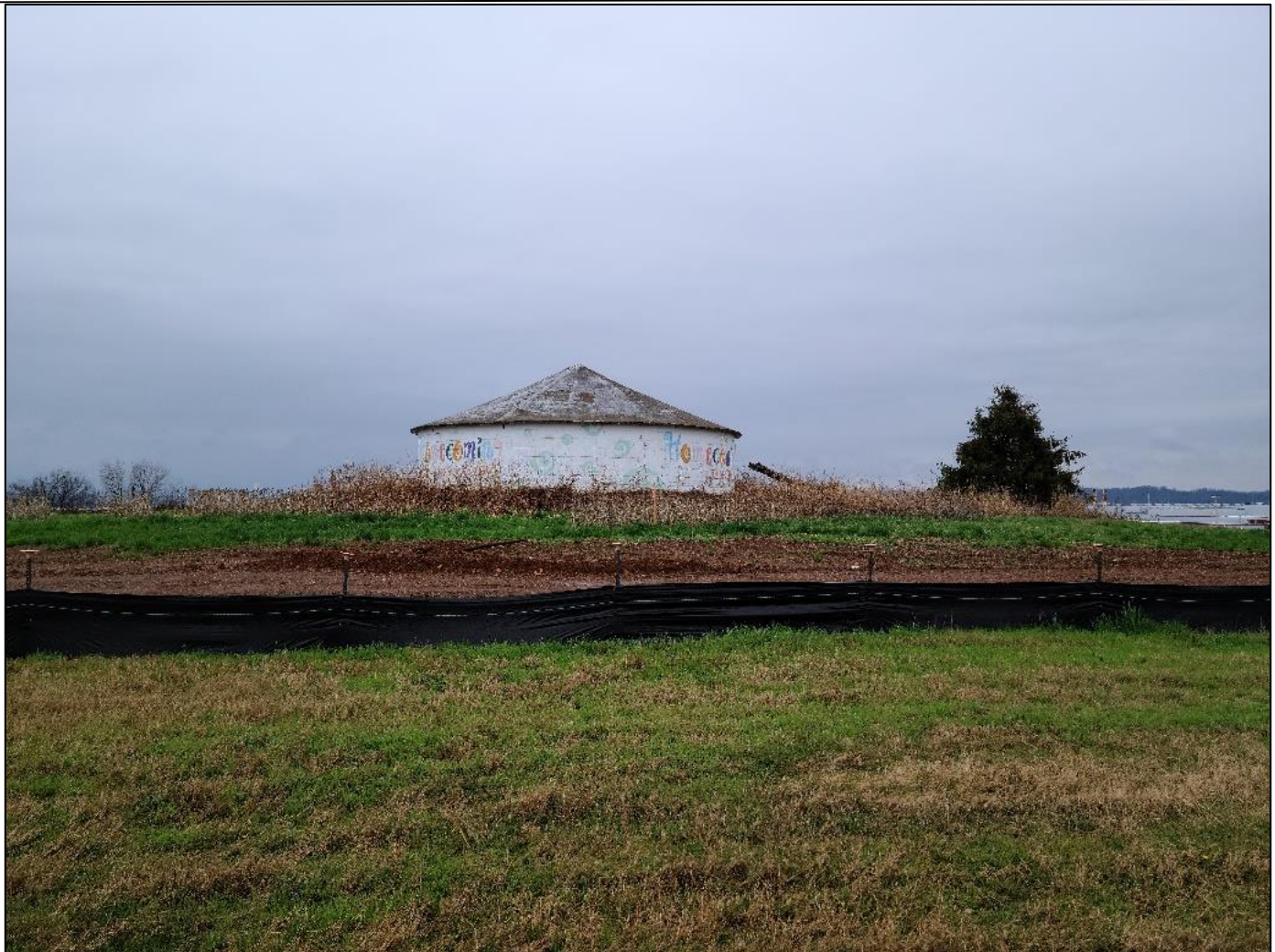
Figure 1. A large concrete water reservoir constructed as part of J. Brice Martin's water supply system circa 1901. Photographed March 15, 2021.
