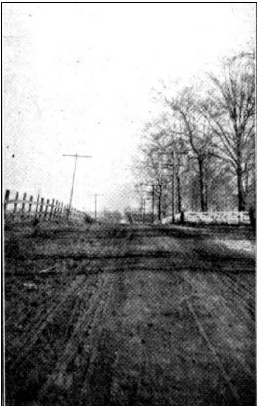
Figure 3. The Columbia and Franklin Pike (later the Nashville and Columbia Pike) in front of Rippavilla near Woodlawn, circa 1906. Trotwood's Monthly , March 1906.
