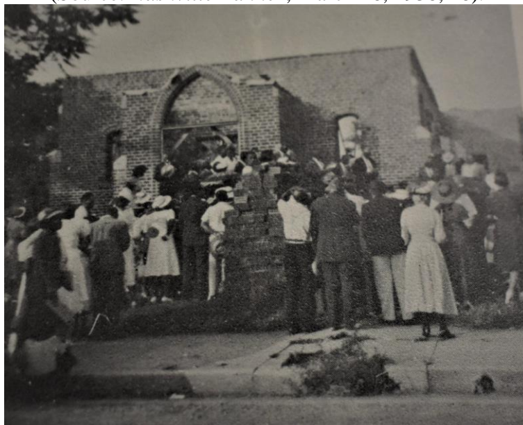
Figure 2. Photograph of the cornerstone laying ceremony, 1942 (Source: Campbelle, “History,” 1967).
