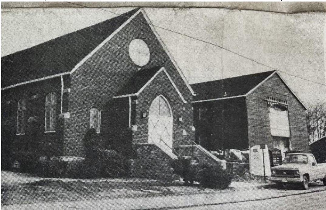
Figure 14. Photograph showing the 1981 wing under construction, circa March 1981 (Source: Clark Memorial United Methodist Church Archives).
