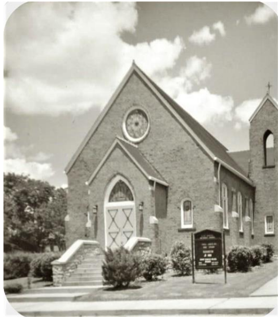
Figure 3. Photograph of Clark showing the sanctuary, 1945 (Source: Stone and Heath, "A Walking Tour," 2017, 3).
