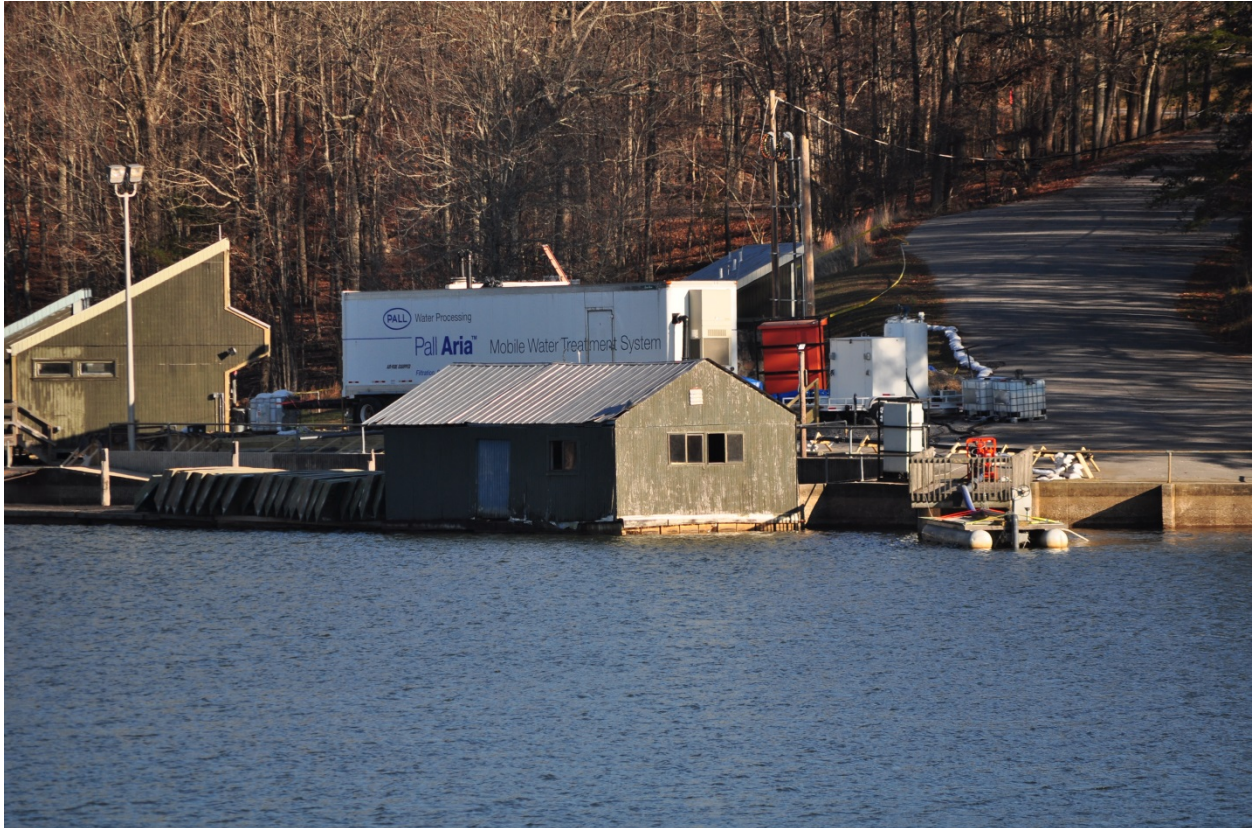
View of the Emergency WTP from the FCFSP Inn
