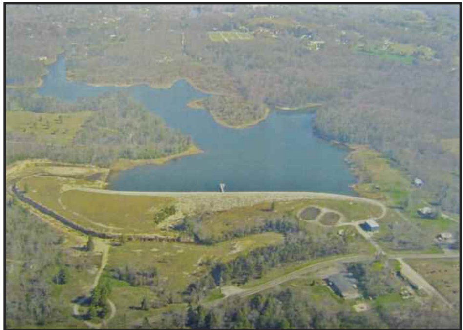
Figure 4-2. Aerial photo of Big Fiery Gizzard Reservoir
