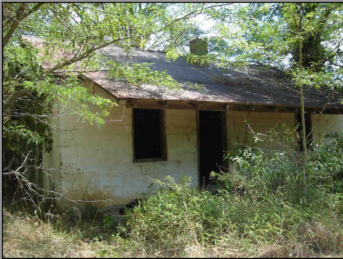
Figure 15. Site 40FY450. View to the Southeast.
