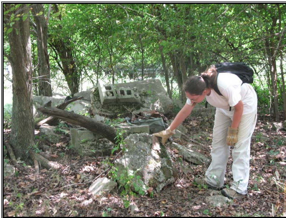
Figure 24. WA-0229-FN2, push-pile. View to the East.
