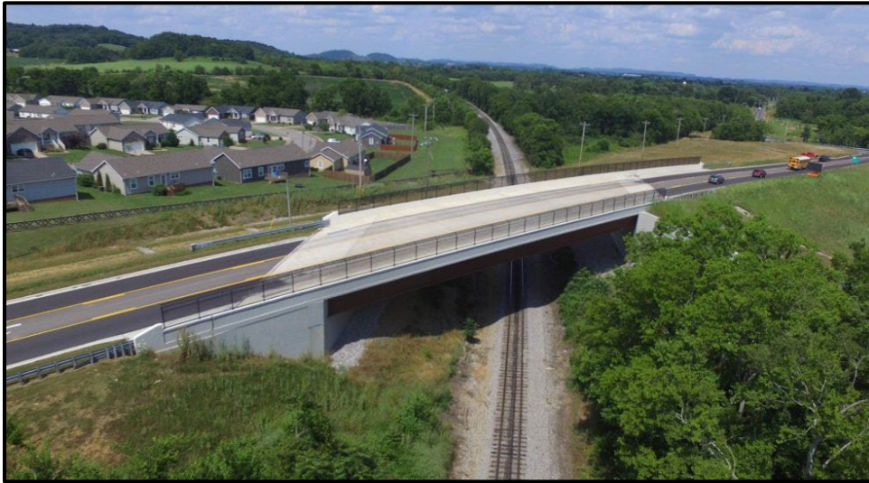
Figure 4-13 Example of Highway over Railroad
