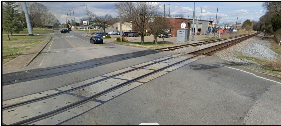
Figure 4-22 Example of an At-Grade Railroad Crossing
