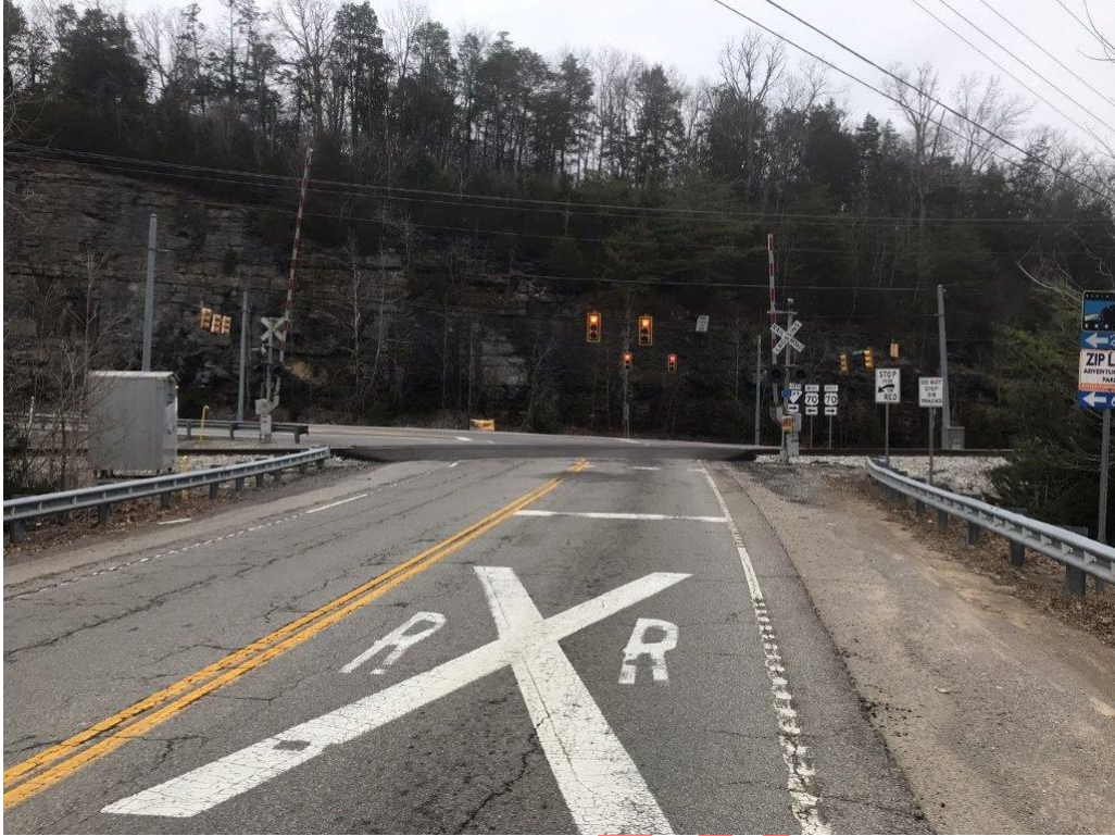
North Approach, E Kingston Spring Rd & HWY 70
