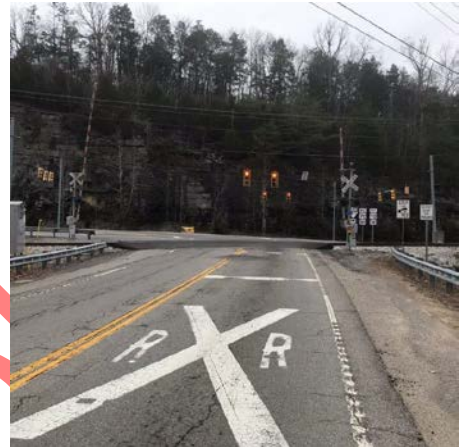
Pavement Marking RxR
