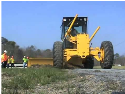
Clipping the shoulder with a motor grader
