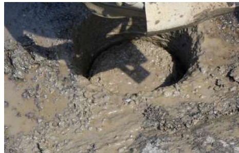
Saturated base/binder layers that strip
