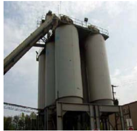
Multiple Surge/Storage Silos
