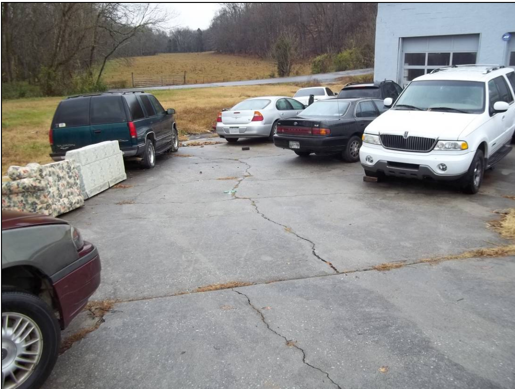
Photo 8: View of portion of Site 5 showing general location where soil boring SB-06 was advanced.
