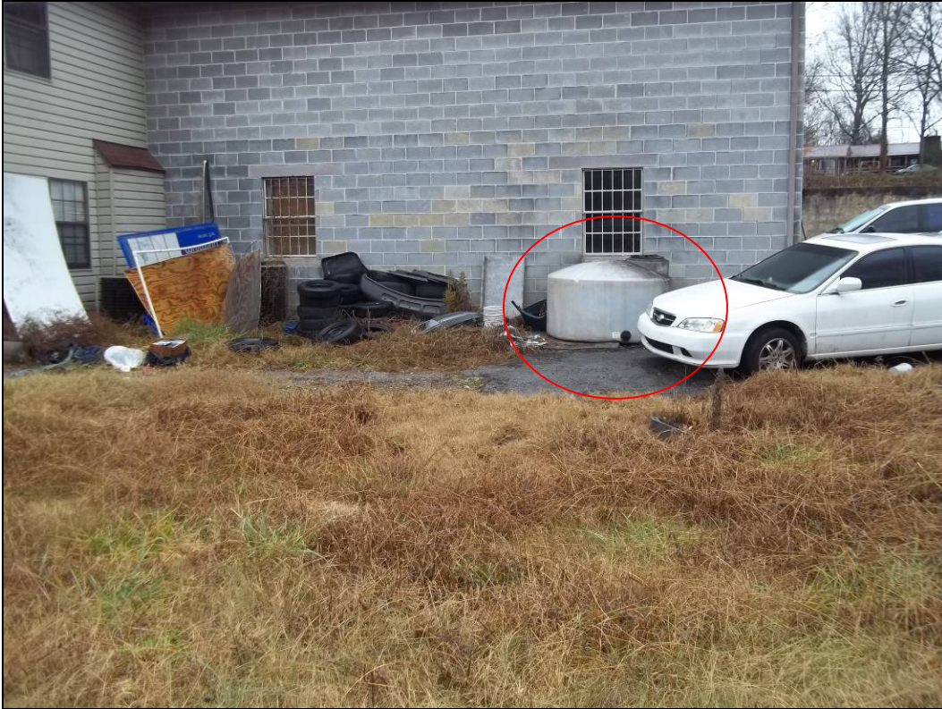
Photo 3: View of portion of Site 5 showing the waste oil AST located behind the building structure.
