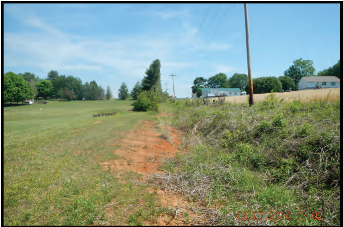
Photo 66 (3177): (Alternative C) Up gradient view of WWC-4.
