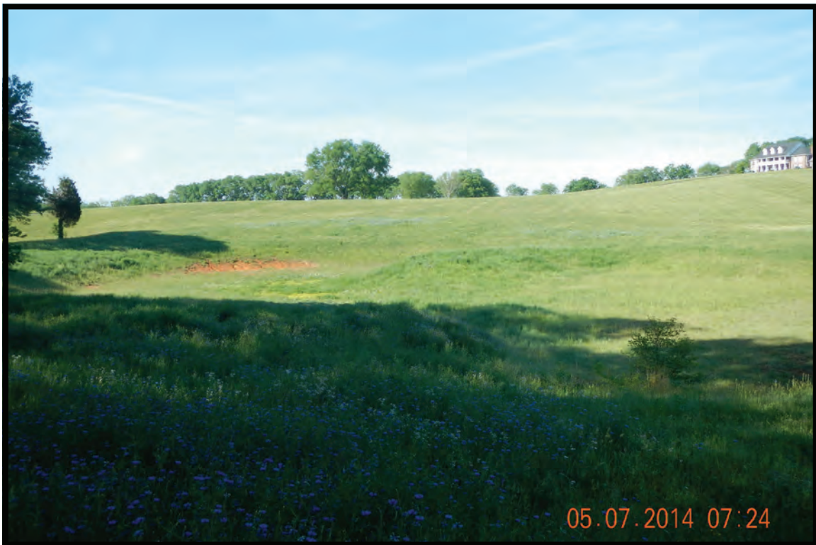
Photo 32 (3143): (Alternative D) View of closed throat sink hole (SNK-1). Feature located west of Sam Houston School Road.
