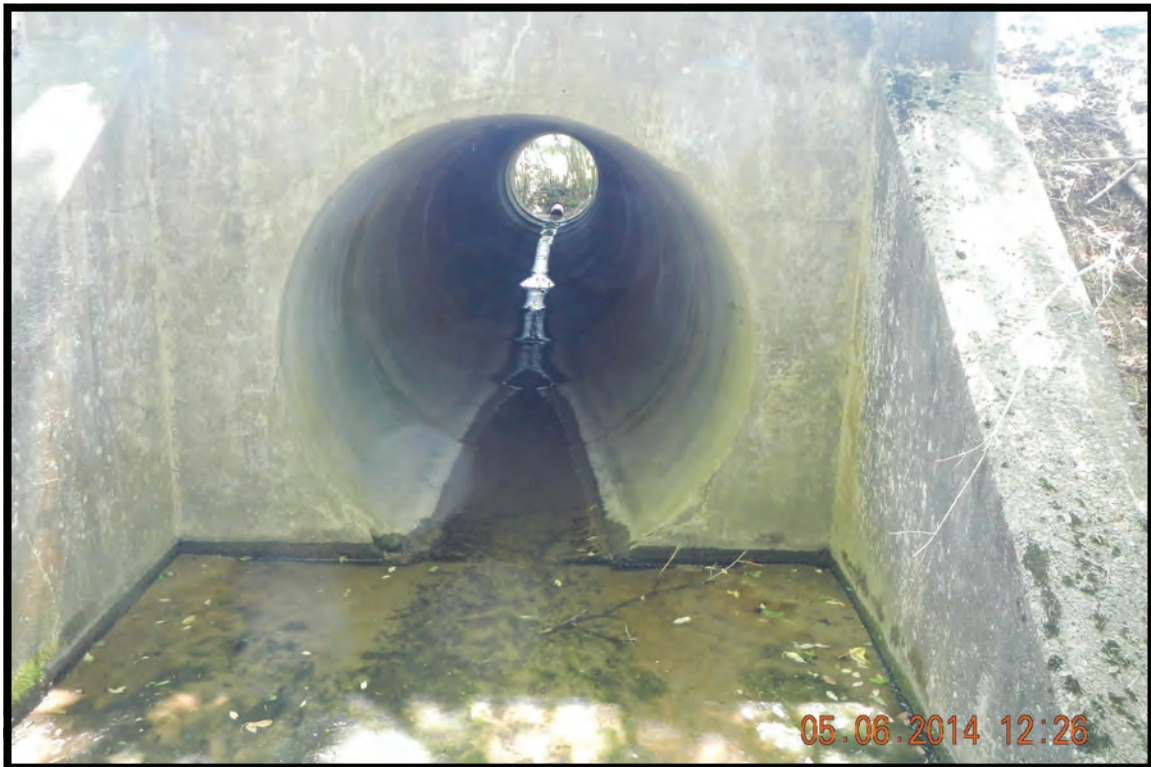
Photo 2 (3112): (Alternative D) Upstream view of STR-1.
