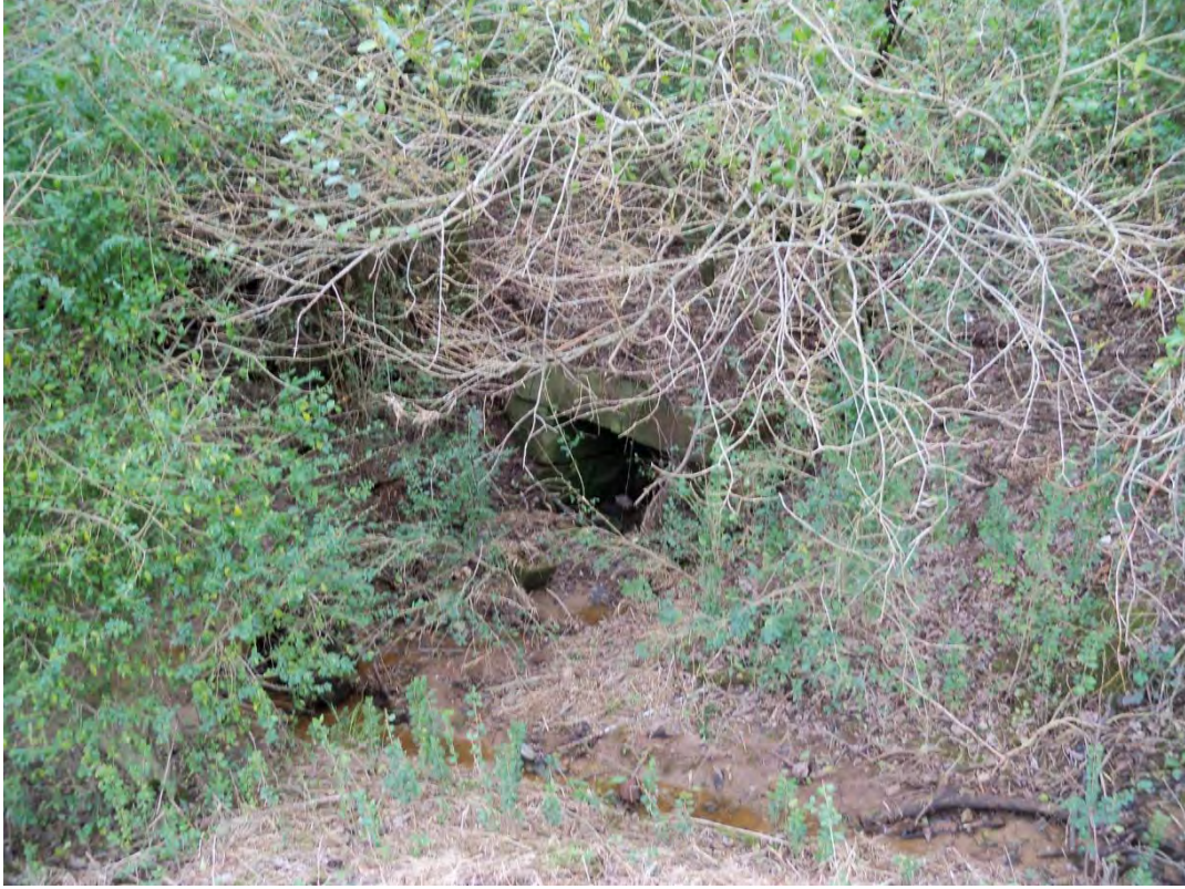
Photo 27: STR-7A View Looking Southeast at north side of railroad bed
