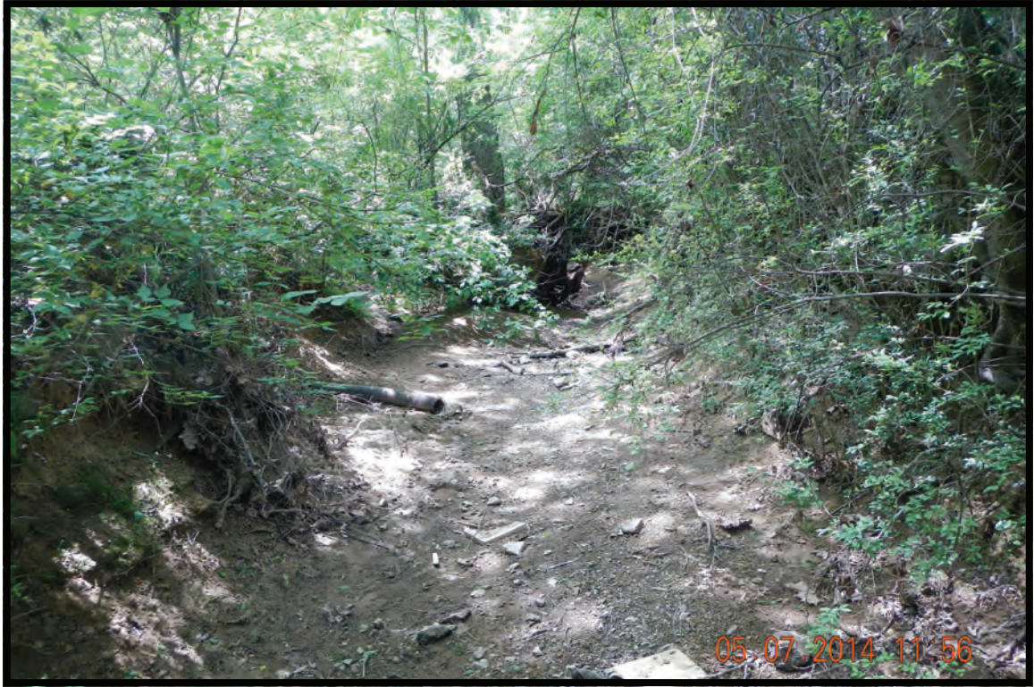
Photo 57 (3168): (Alternative C) Upstream view of STR-3.
