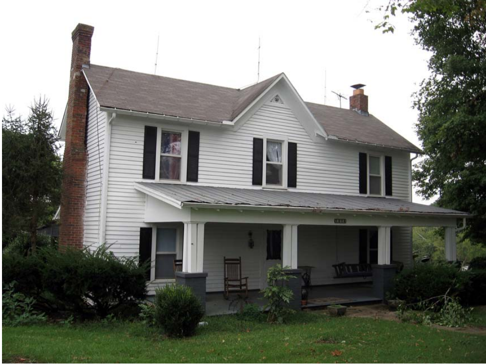
Figure 153. Chandler-DeLozier House looking southeast; the front porch was likely added by George Chandler in the 1920s (R. Jones 9/9/08)
