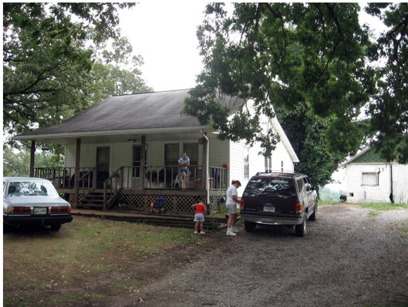
Figure 36. The Archie-Walters House looking southeast (R. Jones 9/9/08)
