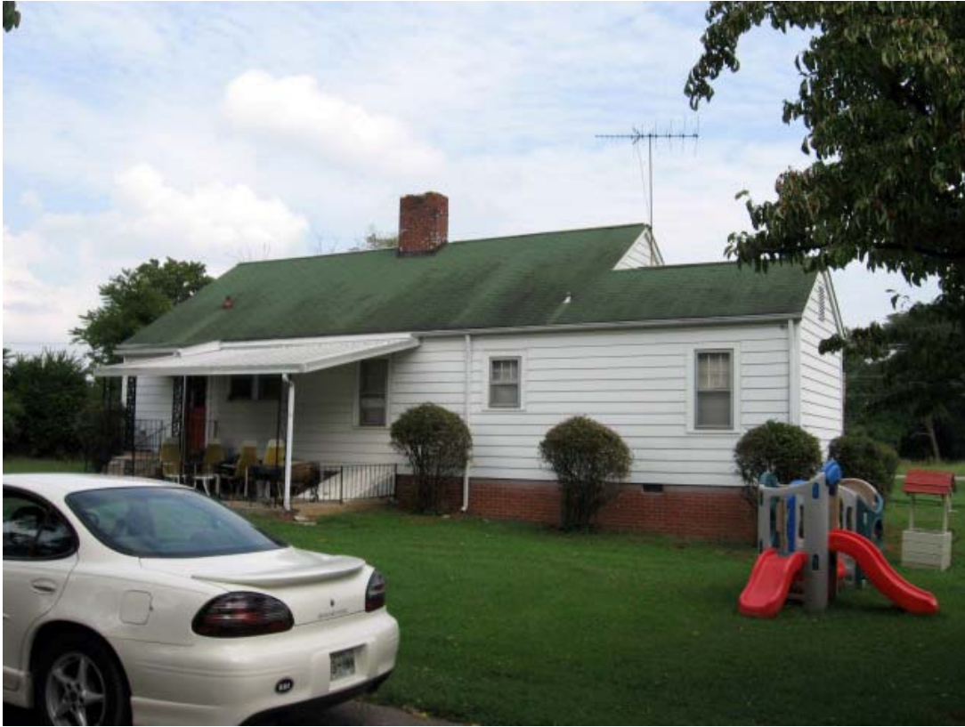
Figure 148. Walker House looking southeast (R. Jones 9/10/08)
