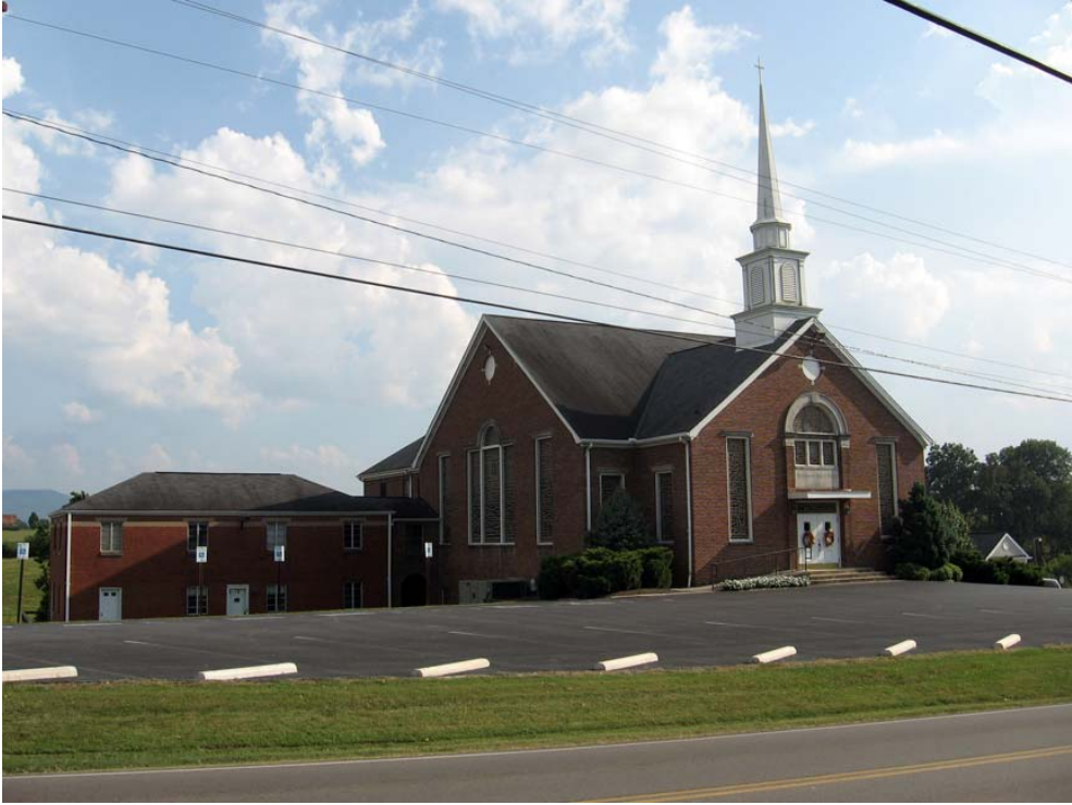
Figure 106. Mount Lebanon Baptist Church looking southwest with the 1948 Education wing on the left and the 1952 sanctuary on the right (R. Jones 9/8/08)
