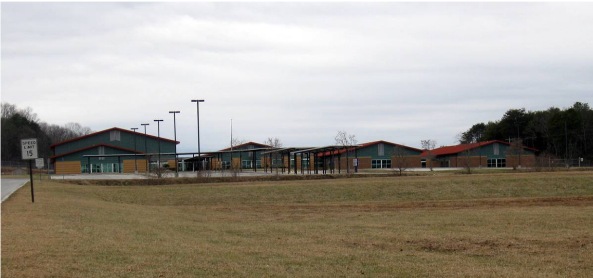
Figure 185. Looking west at the new Eagleton Elementary School located along Sam Houston Schoolhouse road (N. Skinner, 01/17/09)
