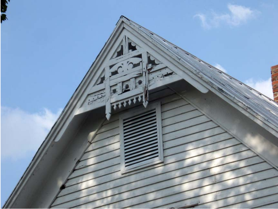
Figure 71. Charles Kennedy House looking northeast at bargeboard trim (R. Jones 9/8/08)
