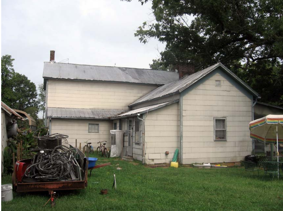
Figure 76. Brown-Keller Farm looking northeast (R. Jones 9/10/08)
