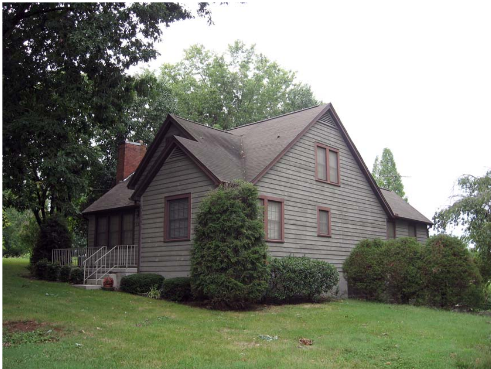
Figure 125. Lynn & Mary DeLozier House looking northwest (R. Jones 9/9/08)
