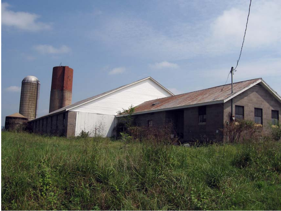
Figure 54. McNutt-Singleton Farm looking east at dairy support buildings constructed of concrete and concrete block in the mid-twentieth century (R. Jones 9/10/08)
