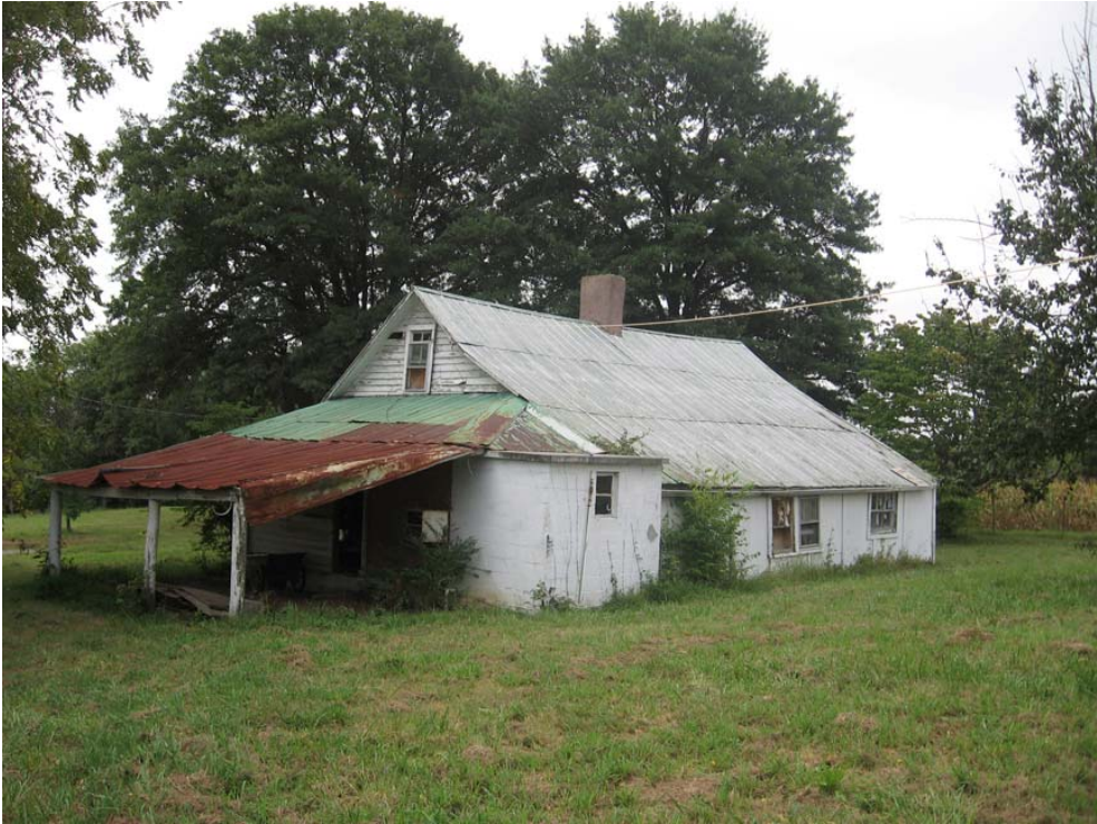
Figure 132. Clyde Irwin House looking southwest (R. Jones 9/10/08)
