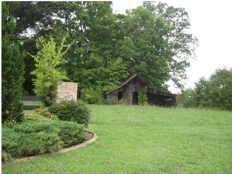
Figure 49. The Chandler-Sharp Farm looking west at the smokehouse (BT.2244) and site of the recently demolished farmhouse (R. Jones 9/9/08)
