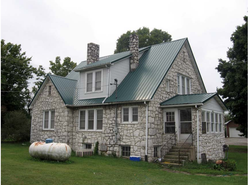
Figure 89. Caughron-Wells House looking south (R. Jones 9/9/08)
