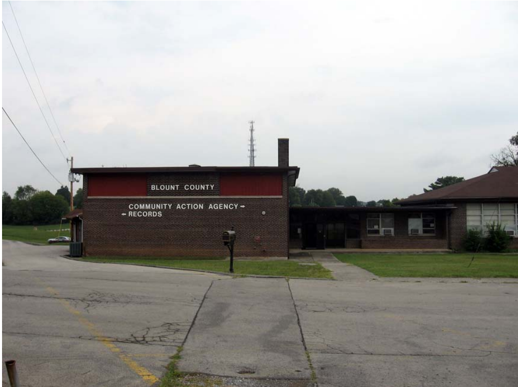
Figure 122. Former Hubbard School looking north (R. Jones 9/9/08)
