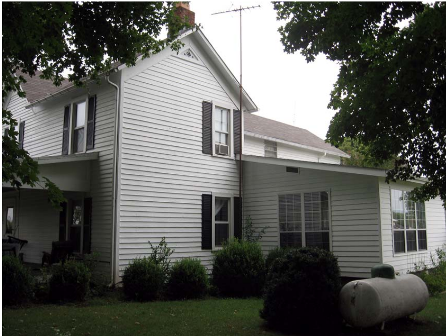
Figure 154. Chandler-DeLozier House looking north; shed addition built by Garland DeLozier in the 1950s or '60s (R. Jones 9/9/08)
