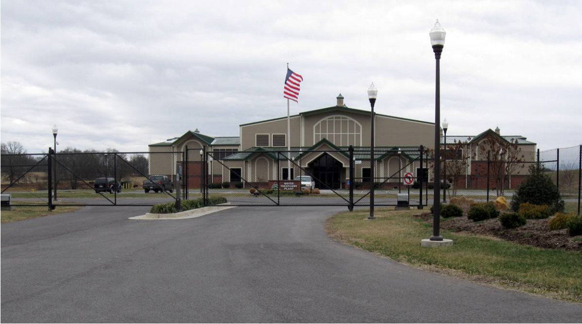
Figure 186. Looking west at the new Water Filtration Plant located along the west side of Sam Houston School Road (N. Skinner 01/17/09)
