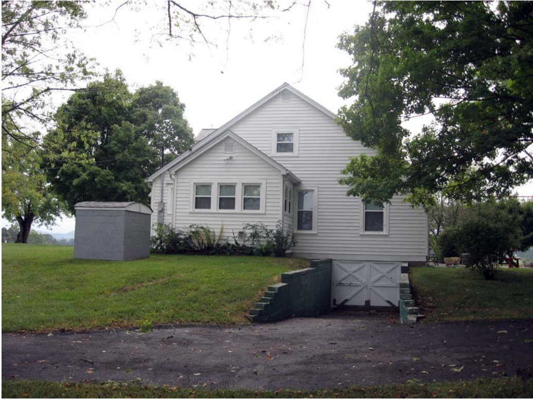
Figure 117. Keeble House looking south (R. Jones 9/9/08)
