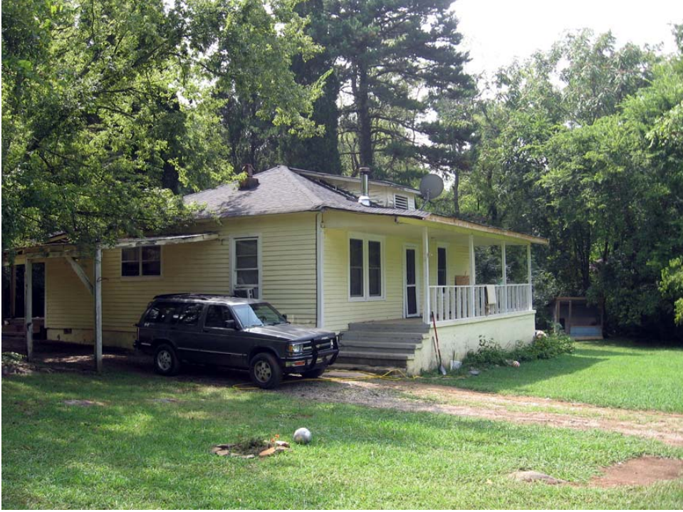
Figure 56. ALCOA House looking southwest (R. Jones 9/10/08)
