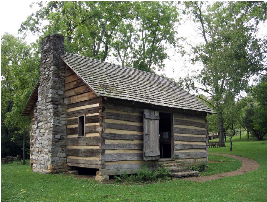
Figure 13. Sam Houston Schoolhouse, looking northwest (R. Jones 9/10/08)
