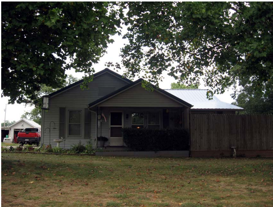
Figure 111. Lem-Morgan House looking north (R. Jones 9/8/08)
