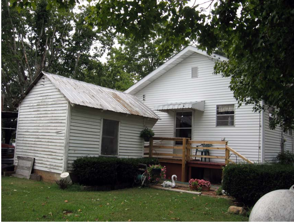
Figure 165. Cusick-DeLozier Farm looking northwest at the rear of the farmhouse and smokehouse (R. Jones 9/9/08).
