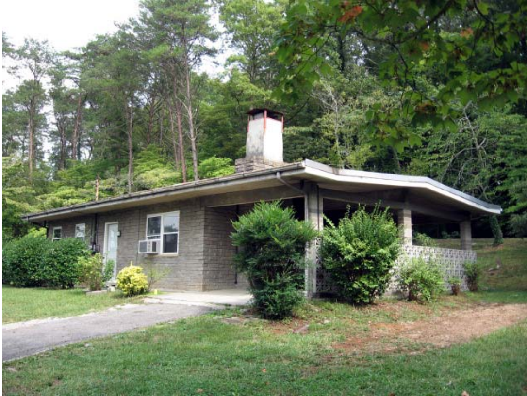
Figure 152. Norton House looking southeast (R. Jones 9/10/08)
