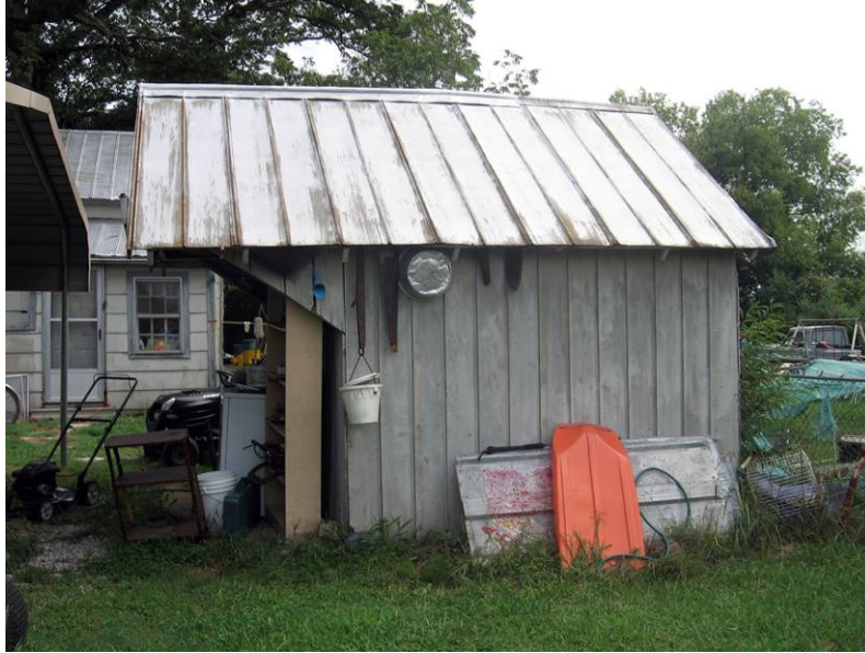
Figure 78. Brown-Keller Farm looking east at the original dairy (R. Jones 9/10/08)
