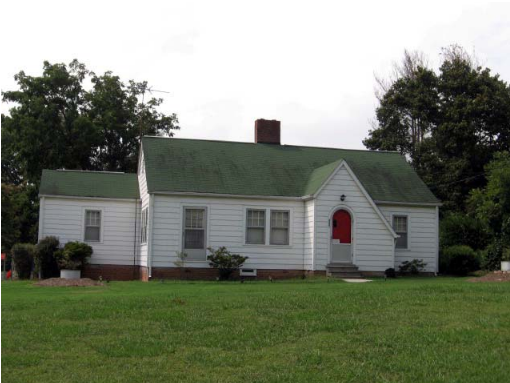
Figure 147. Walker House looking northwest (R. Jones 9/10/08)
