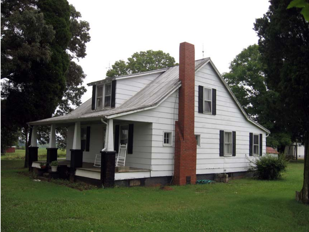
Figure 96. The DeLozier House looking southwest (R. Jones 9/9/08)
