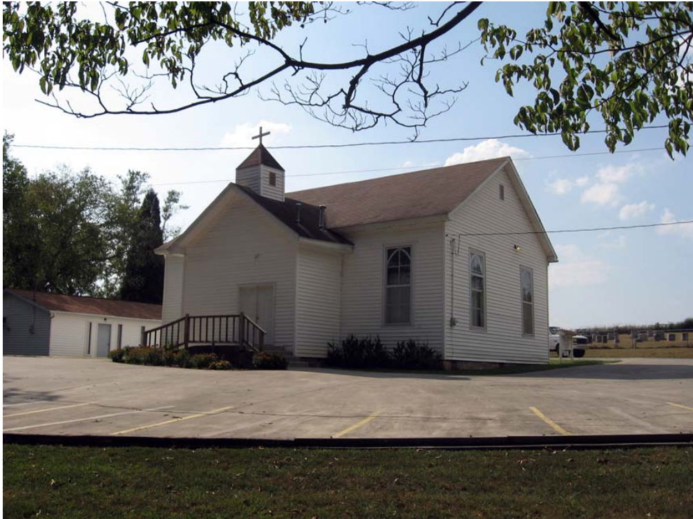
Figure 44. Former Centennial Presbyterian Church looking northwest (R. Jones 9/8/08)
