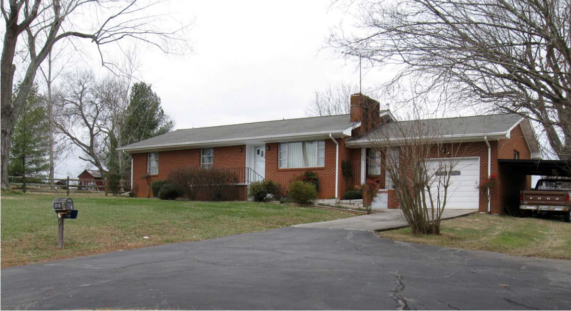
Figure 176. Stafford-DeLozier Farm looking northeast at the Ranch-style dwelling constructed in the 1950s and later enlarged with a garage wing and attached carport (N. Skinner 01/17/09)
