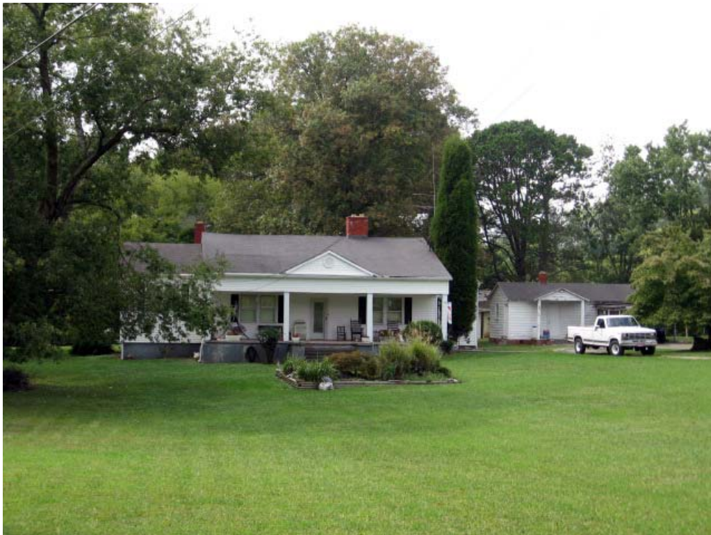
Figure 149. Thames House looking northwest (R. Jones 9/10/08)
