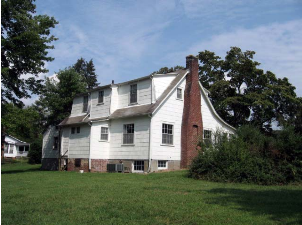
Figure 145. DeLozier House at 3305 Old Knoxville Highway looking northeast (R. Jones 9/10/08)
