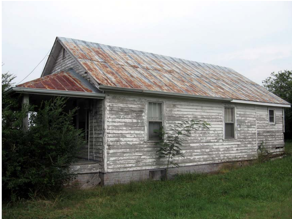
Figure 168. Cusick-DeLozier Farm looking southeast at the 1935 tenant house (R. Jones 9/9/08)
