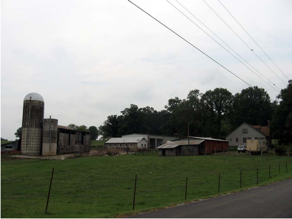
Figure 40. The Martin-Walters Farm looking northeast (R. Jones 9/9/08)
