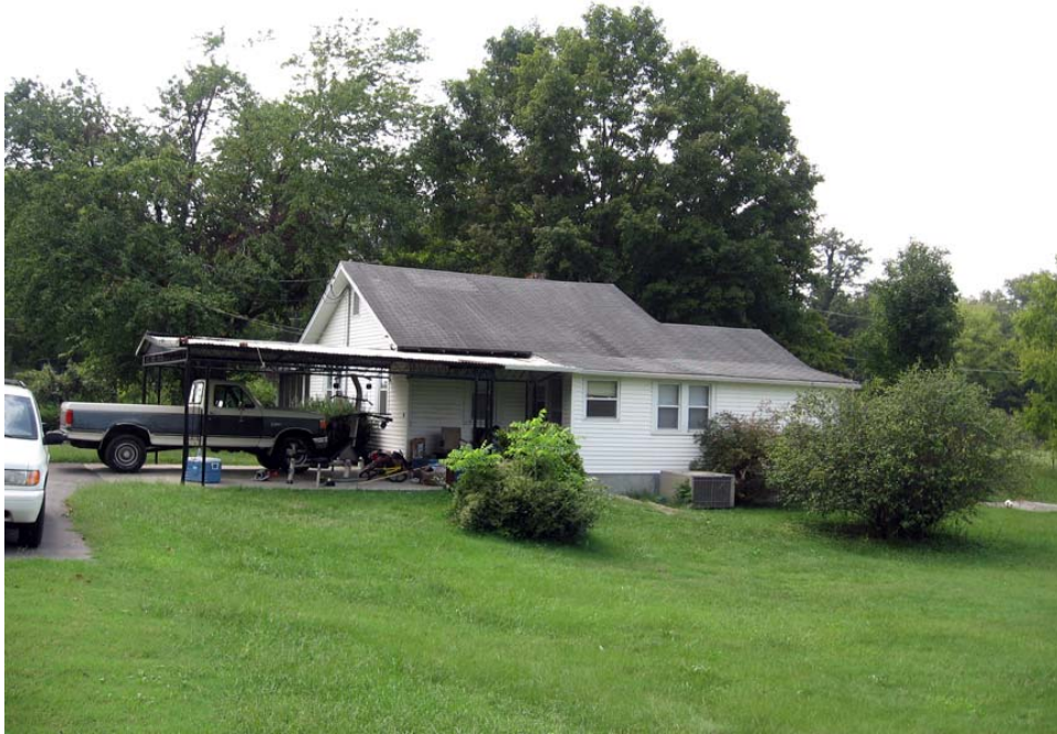
Figure 35. The James & Irene Hitch House, looking southwest (R. Jones 9/10/08)
