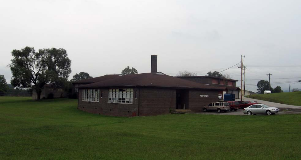
Figure 121. Former Hubbard School looking southeast (R. Jones 9/9/08)
