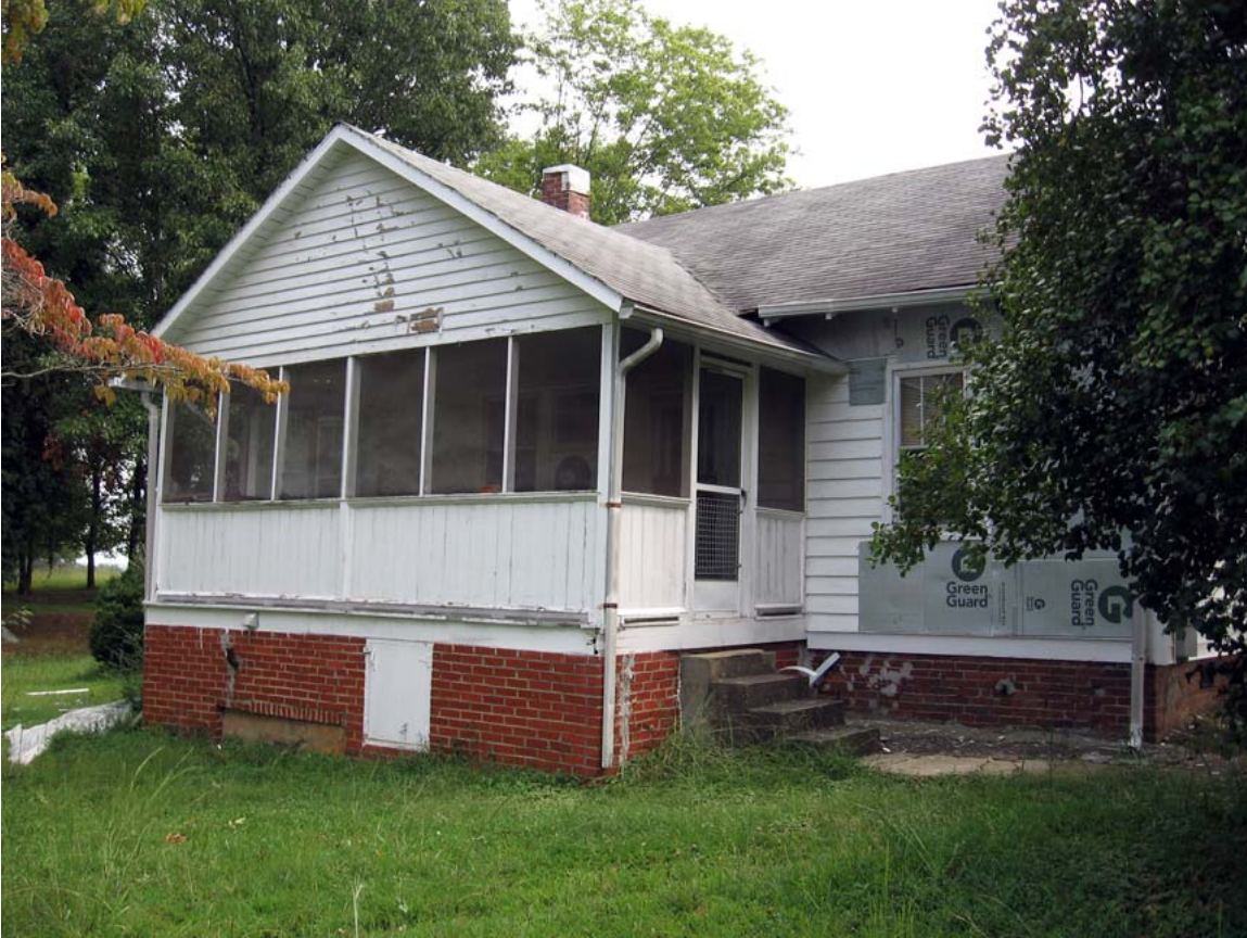
Figure 143. Haddox House looking southeast (R. Jones 9/10/08)
