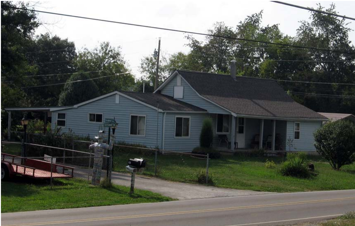
Figure 46. Long-Scarbrough House looking northwest (R. Jones 9/8/08)
