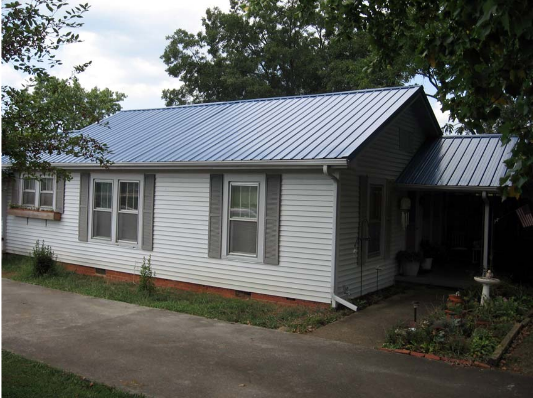
Figure 112. Lem-Morgan House looking northeast (R. Jones 9/8/08)
