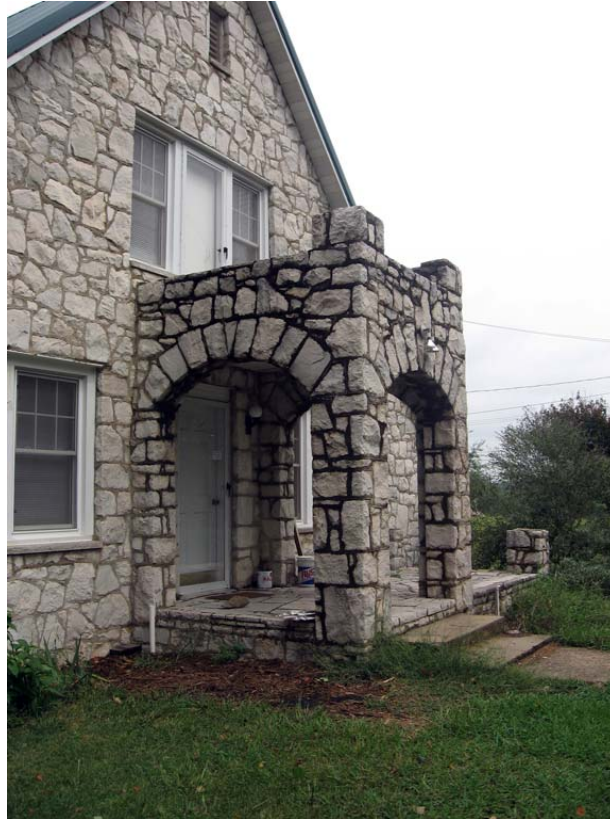
Figure 92. Caughron-Wells House looking northeast at portico (R. Jones 9/9/08)
