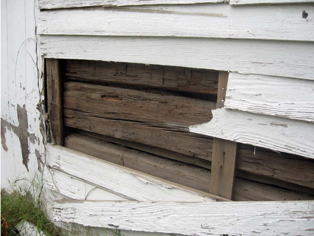
Figure 131. Clyde Irwin House looking northeast at the exposed log walls (R. Jones 9/10/08)
