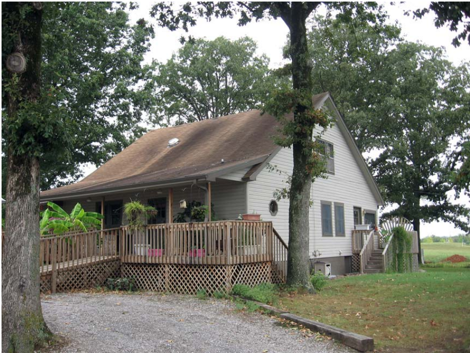
Figure 39. The Martin-Walters Farm looking northeast (R. Jones 9/9/08)
