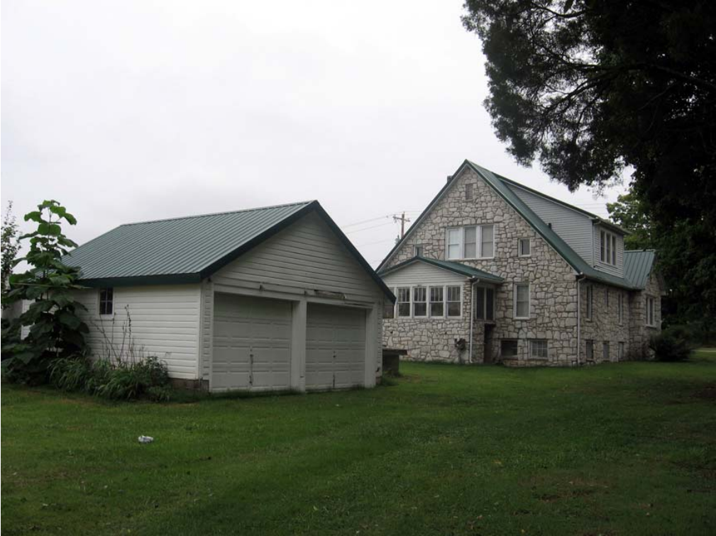
Figure 90. Caughron-Wells House, looking southeast (R. Jones 9/9/08)
