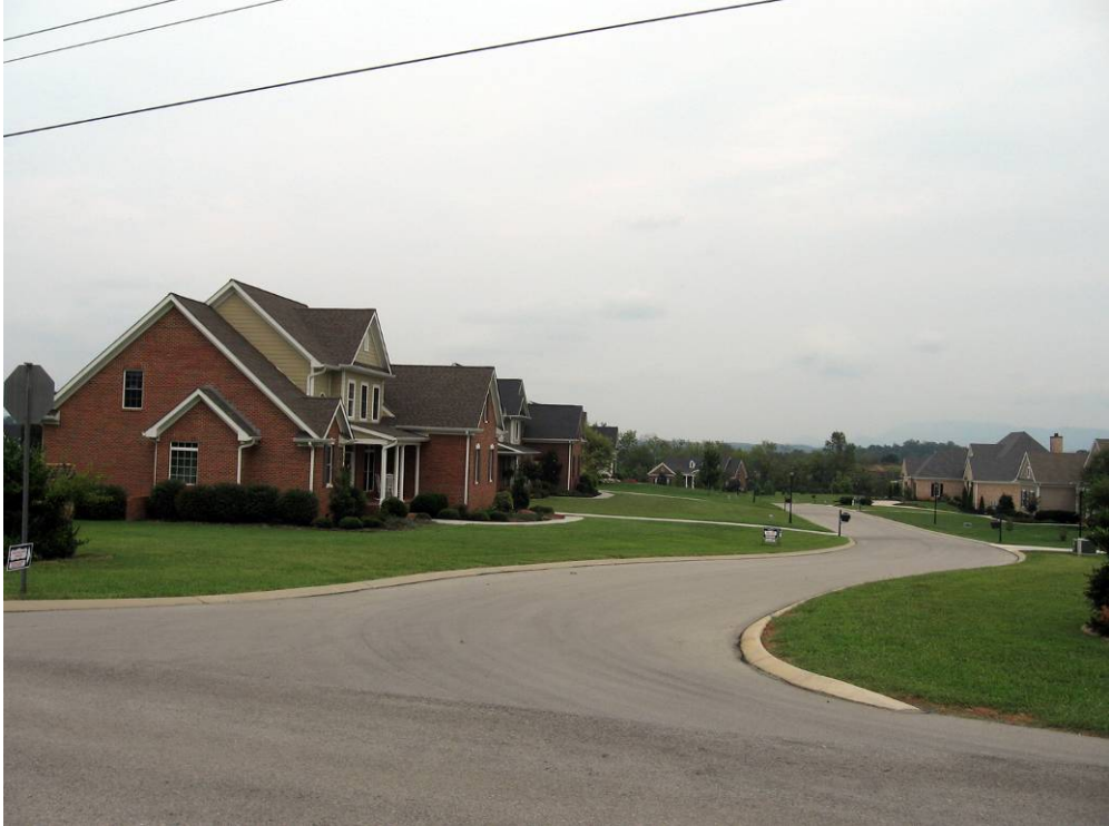
Figure 178. A new residential subdivision, Whittenburg Estates, located on a former farm along Nina DeLozier Road (R. Jones 9/9/08)
