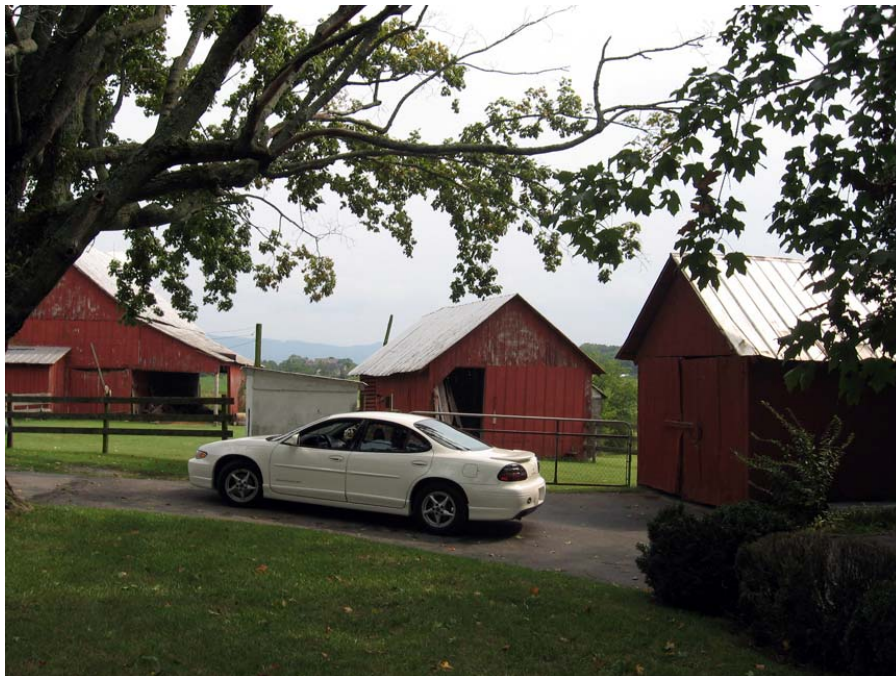
Figure 166. Cusick-DeLozier Farm looking south at the 1918 dairy barn (left), concrete pumphouse (middle left), dairy/crib/shed (middle right), and automobile garage (right); the concrete block dairy is behind the crib/shed (R. Jones 9/9/08).
