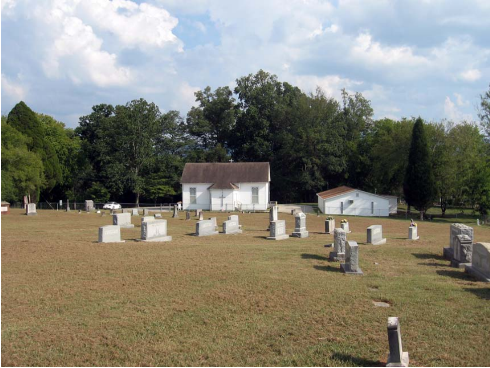
Figure 43. The former Centennial Presbyterian Church looking south from the cemetery (R. Jones 9/8/08)
