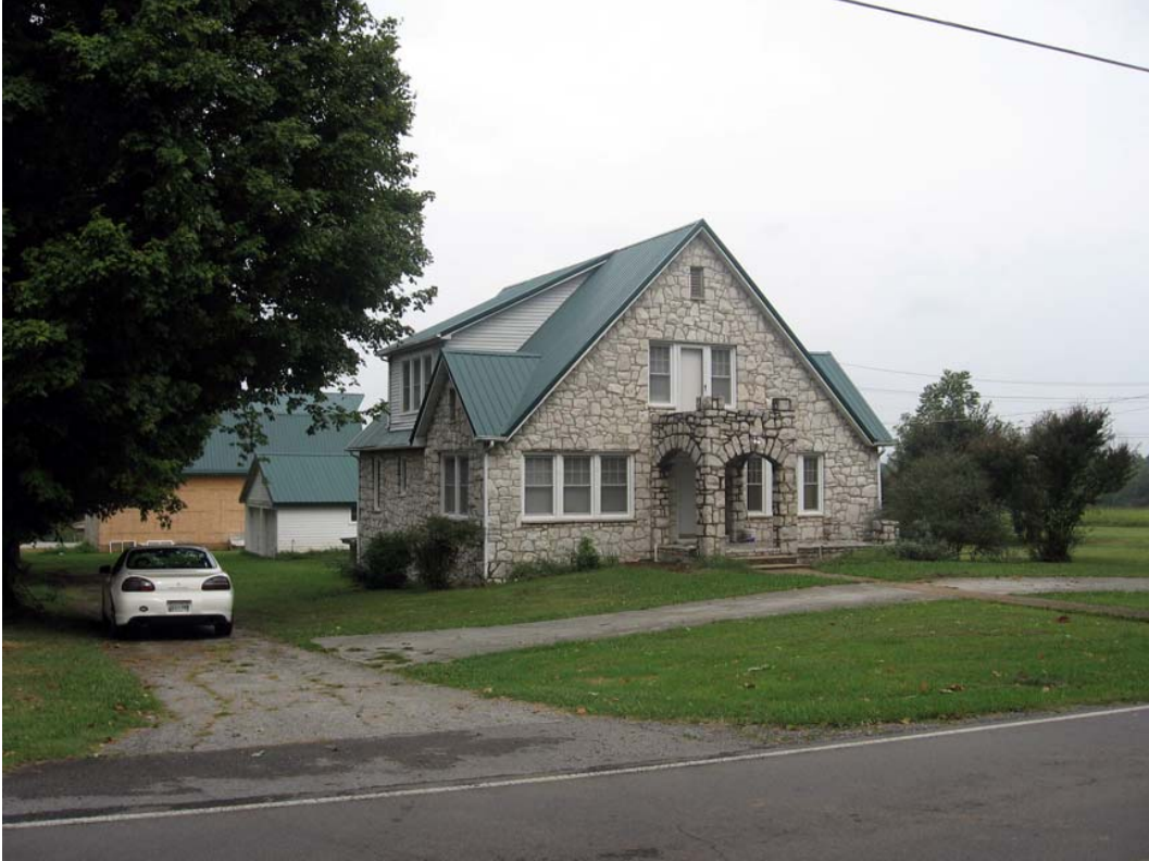
Figure 88. Caughron-Wells House looking north (R. Jones 9/9/08)
