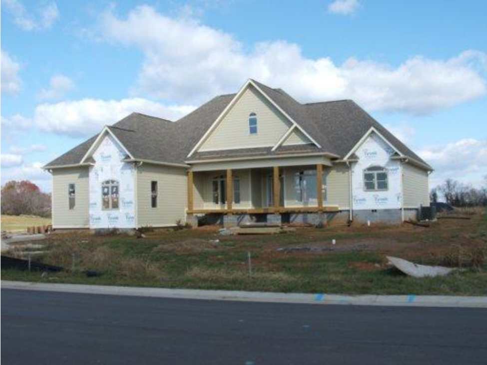
Figure 181. A new home under construction in 2008 at Sweet Grass Plantation.
