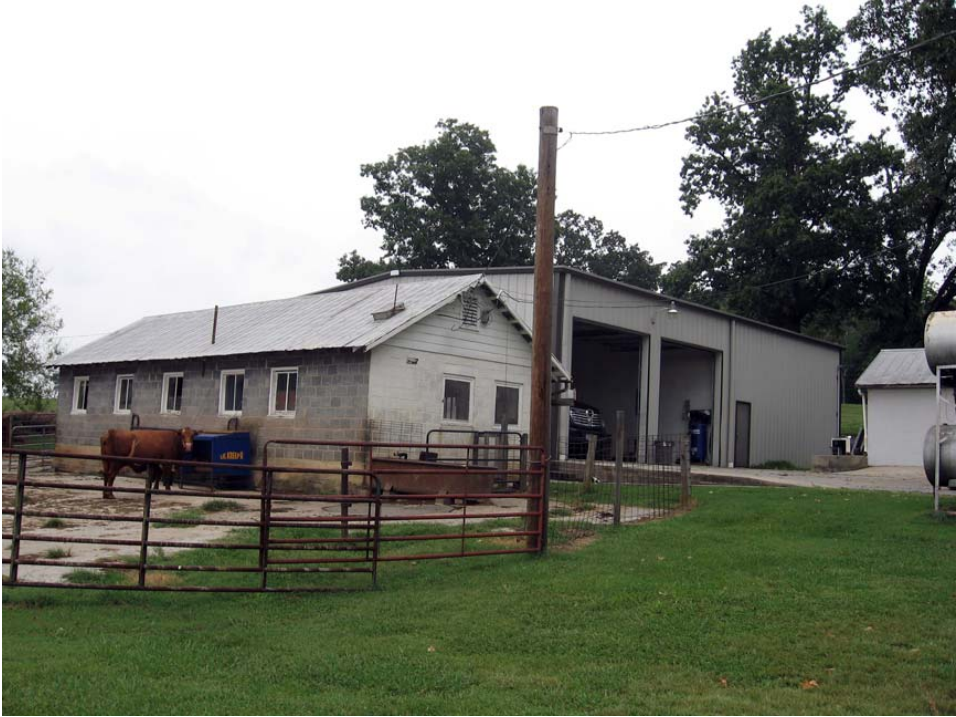
Figure 41. Martin-Walters Farm looking northwest at the Bulk Milk Cooler (left) and the modern truck garage (right) (R. Jones 9/9/08)
