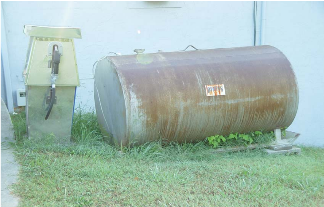
Site No. 5 – View showing kerosene AST.
