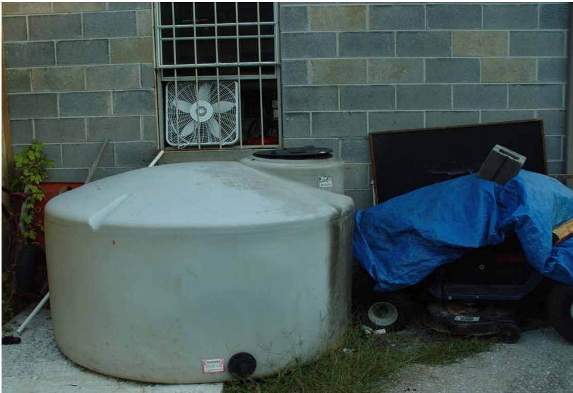
Site No. 5 – 550-gallon used oil AST.
