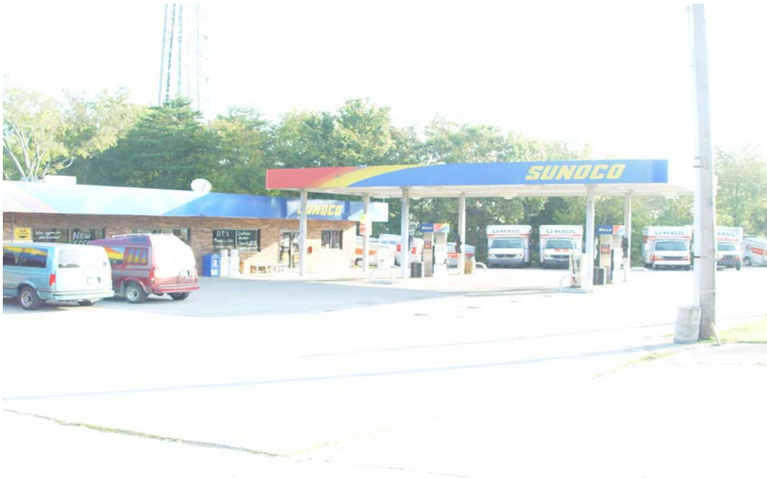
Site No. 4 – View showing store and fuel dispensing island.
