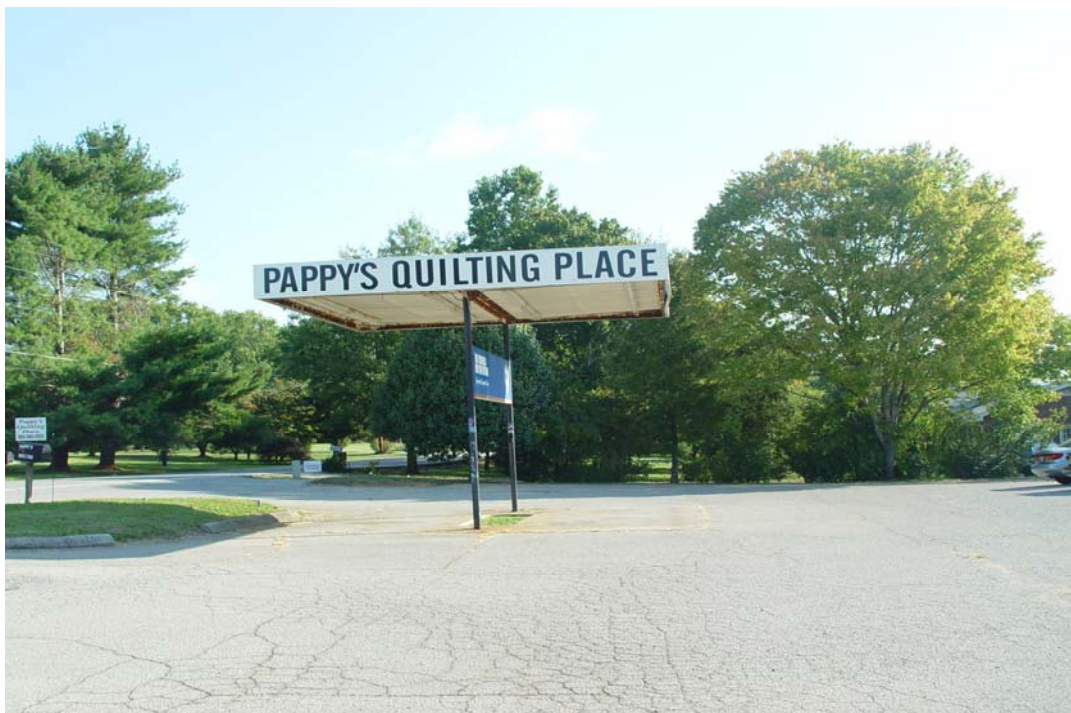
Site No. 2 – View showing former fuel dispenser island.
