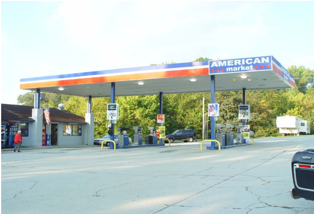
Store No. 5 – View showing store and fuel dispensing island.
