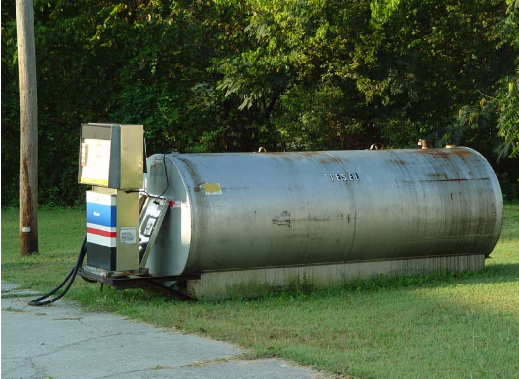
Site No. 5 – View showing diesel fuel AST.
